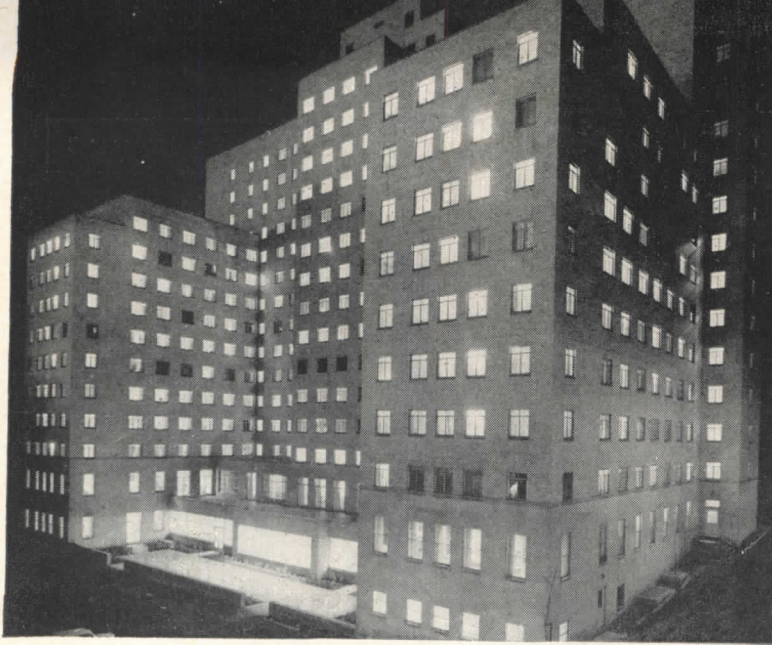
The $3.5-million nurses home at University of Pittsburgh towers 14 stories, completely air conditioned, contains library, recreation room, reception rooms, cafeteria seating 400—comfortable living quarters for 600. Steeltex in upper floors. Ingham, Boyd & Pratt, Architects. Trimble Company, Contractors.
