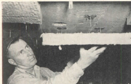
Insulating Walls and Ceiling by Miracle Surface Anchor Method. Fiberglass insulation, Type PF-613, 2" thick — bonded to concrete ceiling using Miracle Pronged Anchors. (Illustration: Radio City Studio 3B, New York, N. Y. Contractor, William J. Scully, Inc., New York, N. Y.)
