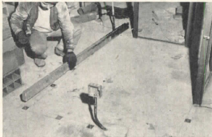
Installing Floor Runners or Bonding Furring Strips. Wood runners installed on concrete floors with Miracle Adhesive and Miracle Anchor Nails to support 2" solid partitions. (Illustration: Washington Circle Apartments, Washington, D.C. General Contractor, Charles H. Tompkins Company.)
