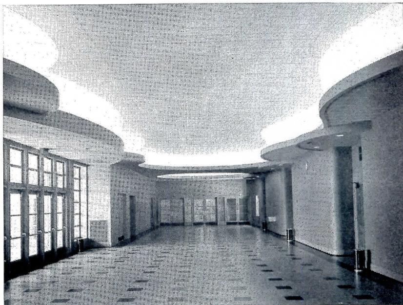
Easily washed or repainted, Cushiontone ceilings in the corridors are simple to keep clean and new looking. A perforated, white painted fiber tile material, Cushiontone soaks up noise efficiently, economically.
