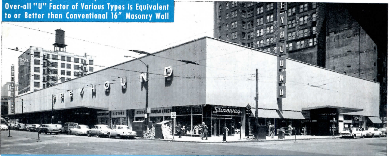
New Greyhound Terminal, Chicago, Illinois. 17,200 Sq. Ft. of Mahon Stainless Steel Metal Walls were employed in exterior surfaces. Skidmore, Owings & Merrill, Architects. John W. Harris & Associates, General Contractors.
