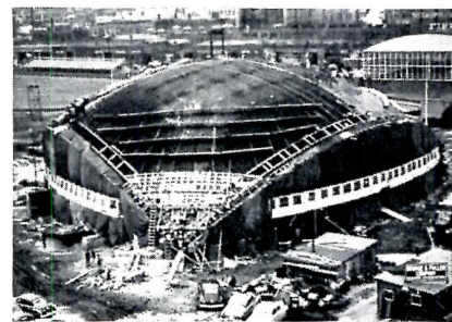
1. Formwork partially completed. Edge beam forms were erected, then timbers forming concentric rings, followed by stringers from bottom to top. 2. Matched lumber was nailed to stringers to receive concrete. 3. Reinforcing in place. 4. Double forms with ports were used on steep slopes near supports; above these forms are platforms for workers. Below: the dome after stripping of forms
