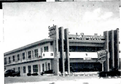
SANDY SHORES Geo. Winston Construction Co.
