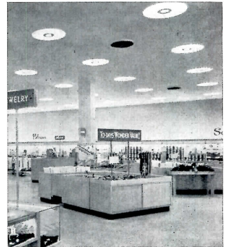
Uniform general lighting combined with valance and shelf-rack lighting prevents a flat, monotonous appearance. Photo, left, shows effect with overhead lights off; photo, right, all lights on. Lerner's, New York City. Cordes, Bartos and Minhos, Architects
