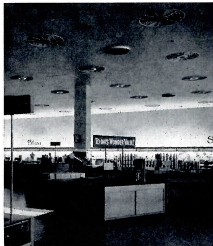
Uniform general lighting combined with valance and shelf-rack lighting prevents a flat, monotonous appearance. Photo, left, shows effect with overhead lights off; photo, right, all lights on. Lerner's, New York City. Cordes, Bartos and Minhos, Architects
