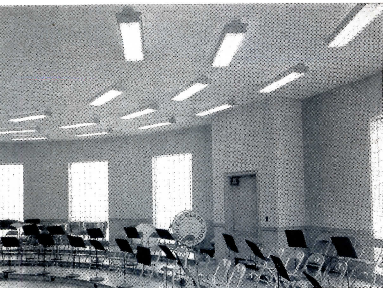
In the band room, sound-absorbing Cushiontone covers the ceiling and upper walls. This acoustical treatment helps prevent build-up of distracting noise levels and provides proper acoustics.
