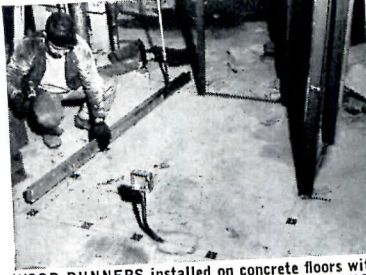
4. WOOD RUNNERS installed on concrete floors with MIRACLE ADHESIVE and MIRACLE ANCHOR NAILS to support 2" solid partitions. Washington Circle Apartments, Washington, D.C. GENERAL CONTRACTOR, Charles H. Tompkins Company.
