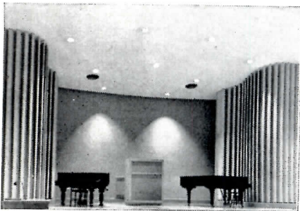
Stage of music auditorium is lighted with 32 recessed incandescent units shielded with PYREX brand Lenslites.
