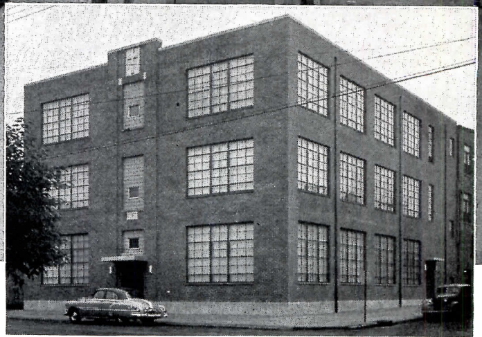
Classroom view, Our Lady of Mt. Carmel School. Tru-Perimeter Heating with Webster Walvector. Sleeves in columns between windows simplify piping without loss of structural strength.
