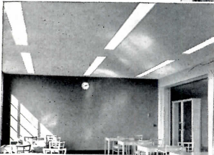
Classrooms, assembly hall, and corridors feature recessed fixtures also shielded with Alba-Lite low-brightness lightingware.
