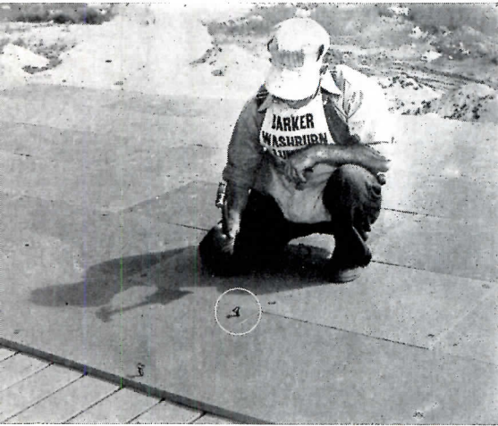
Left: fire-retardant roof uses special clips (above) to apply insulation without mopping to steel deck
