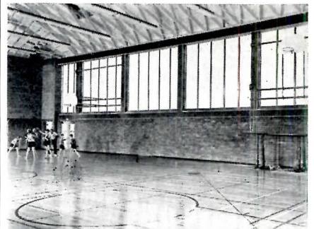
Shatterproof windows used in gym
