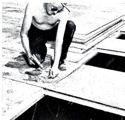
Left: a continuous fabricating process used for Tectum panels. Below: typical roof installation
