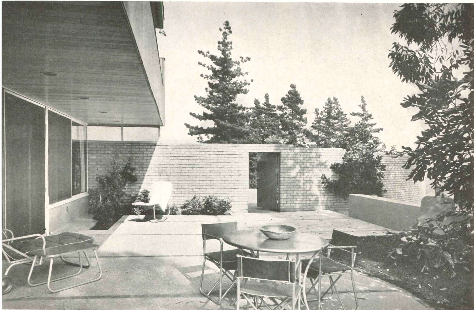
Terrace overlooks the city — but distantly, over the trees. Paving is cement with exposed aggregates and brick liners
