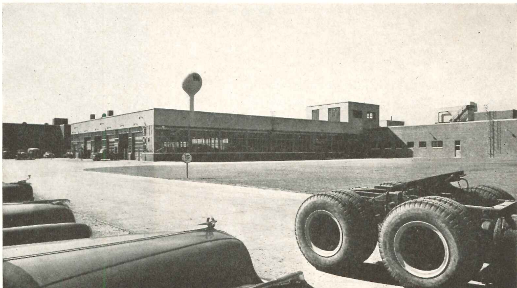
Courts between the wings of the E-shaped building prove useful for access to various sections and parking space for the trucks under study, also for exterior display purposes. Entire building was placed on fill of silty blue clay compacted by sheepsfoot rollers
