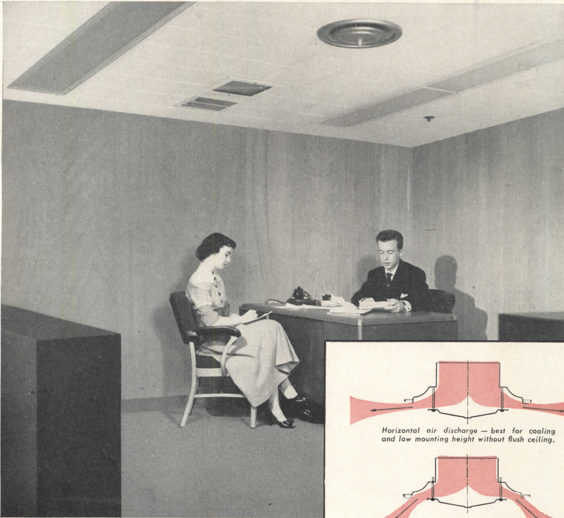
Moderate downward air discharge — best for average conditions.
