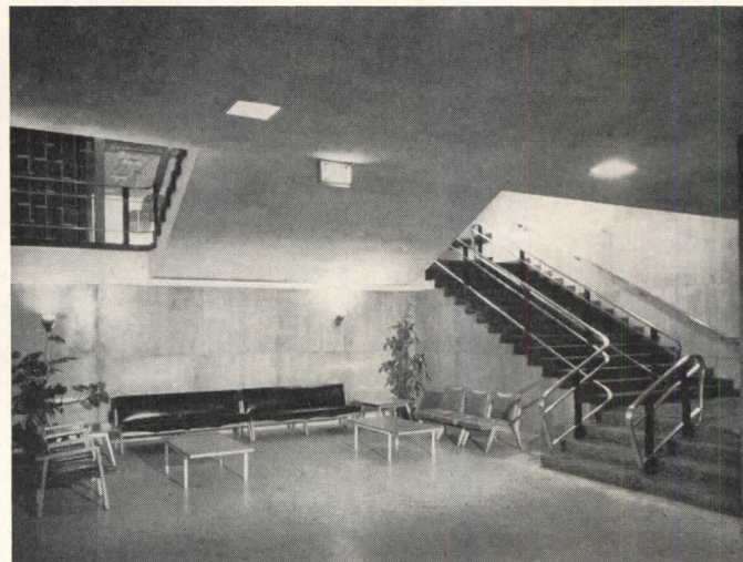
Principal stair has terrazzo treads and risers, satin-finished aluminum handrails, ends at ground floor level in lobby for ballroom
