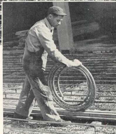
GUIDE PLANK is used by workman to facilitate installation of 1" Type K soft temper Revere Copper Water Tube. Revere Tube also comes in hard and soft tempers in straight lengths of 20 ft.
