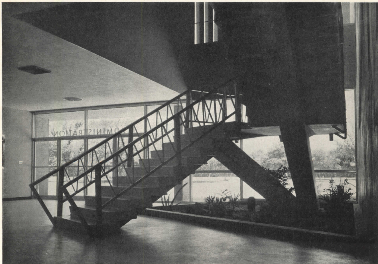
Photo above and on left page: spandrels and corner towers of buff brick—exterior stair of reinforced concrete, interestingly cantilevered from a central column—fireproofing for exterior steel columns of precast rather than poured concrete—all exterior metal aluminum, including sash and entrance doors. Below: stair in administration wing lobby is reinforced concrete with terrazzo finish, aluminum rail
