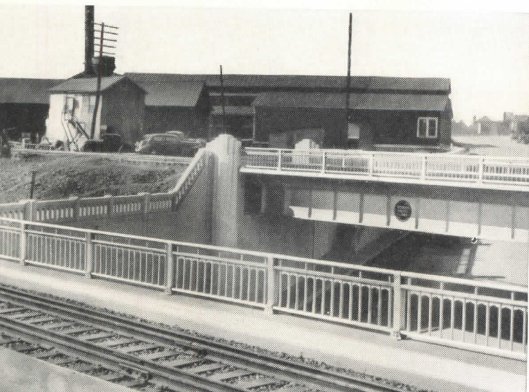
Railings of Alcoa Aluminum on this Little Rock, Ark., railroad bridge have stood up through fifteen years of smoke and soot; never needed paint or upkeep.
