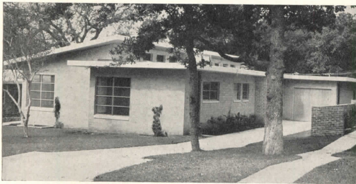
An all-ceramic house under test at The University of Texas can maintain lower daytime temperatures by utilizing night air to cool down the walls, which will then soak up daytime heat
