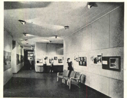
Adjustable spotlights in dual-purpose installation at Pratt Institute, New York
