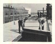
Notched, precast slabs feature light weight, rapid erection, durability
