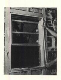
rigidity. The panels are claimed to have excellent thermal qualities, to be moisture proof and to be sufficiently rigid. The moldings are of metal, surfaced with plastic of the same design, color and texture as the panels, to help conceal joints. The molding is nailed to studding to hold panels in place.
