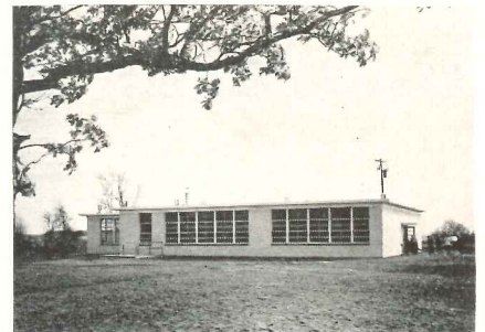
First unit of expandable school is equipped with heater to serve next addition
