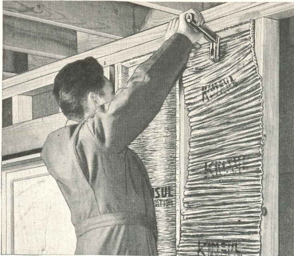
1 Required length of KIMSUL* blanket is cut from roll and stapled to top plate through fiber strip.
