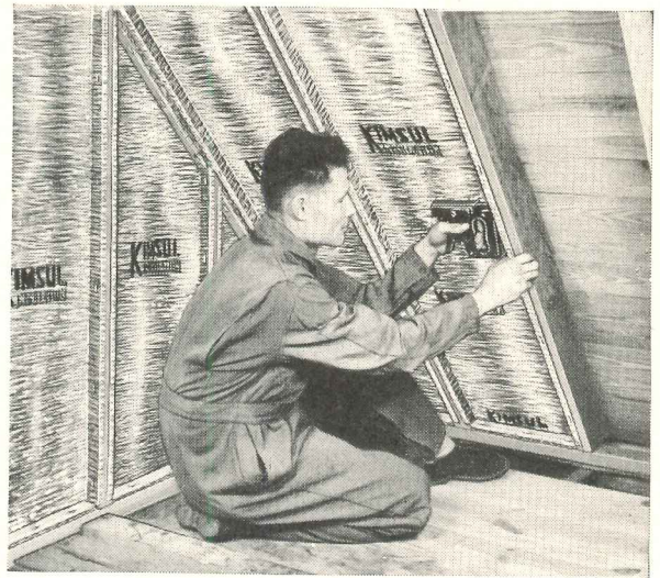
4 Flanges stapled to sides of framing hold blanket permanently in position and also provide air space. Part of flange folds over face of framing to complete vapor seal.
