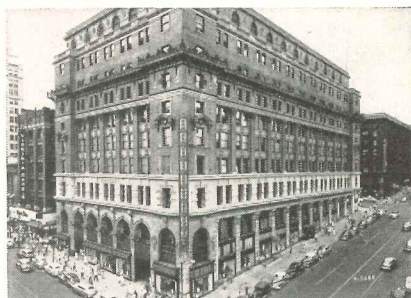
J. L. Brandeis & Sons, Omaha, has installed a Worthington 67C98 centrifugal refrigeration system (647 ton capacity) for air conditioning the lower floors of this store building. Engineering by Charles S. Leopold Company
