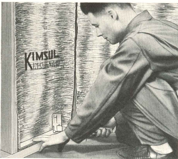
3 Staples through fiber strip attach end of KIMSUL blanket securely to floor plate. Stitched construction assures uniform coverage—prevents thick spots, heat-leaking thin spots.
