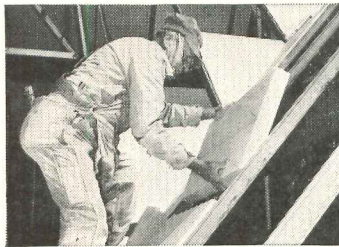
Photograph shows application of Kaylo Roof Tile to a new dormitory of the University of Tulsa, Tulsa, Oklahoma. Architect—Atkinson & Murray. Contractor—Al Ward Construction Co.
