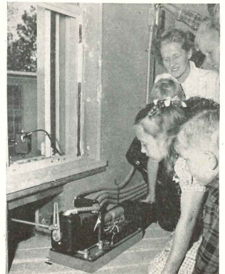
Vertical louvers in new school (above) are automatically operated by photo electric cell and motor. A single master louver controls the entire bank (below)
