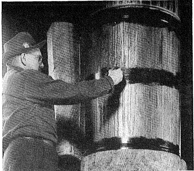
Fiberglas Aerocor* is an exceptionally light weight, highly resilient, blanket-type insulation especially suited for round or irregularly shaped ducts.
