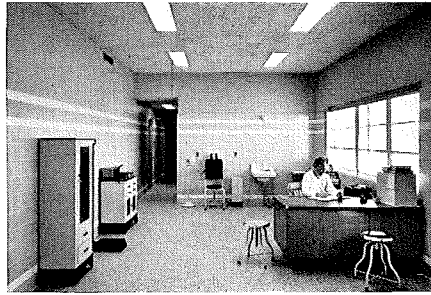
First building in from the main entrance is the time and pay office, housing payroll, employment and personnel offices, also a complete first aid station for workers
