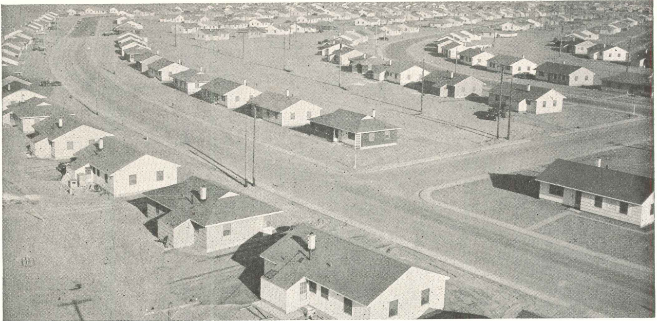
EACH OF THE 1000 HOMES in the Richland, Washington, Housing Project has aluminum heating ducts throughout. Central
