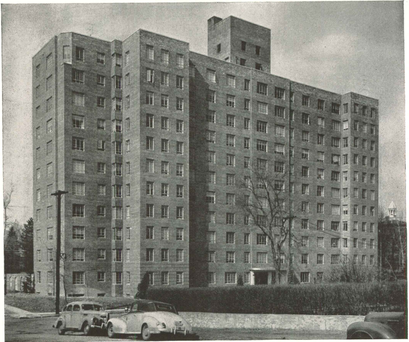
Architect: Rosario Candela, New York. Engineer: Louis d'Antona, New York. Steel Fabricator and Erector: Schacht Steel Construction, Inc., New York.
