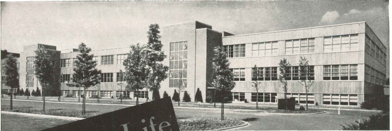
New building addition to Country Life Press, Garden City, N. Y., containing 110,000 sq ft of floor space with electrical raceways always quickly and conveniently available.
