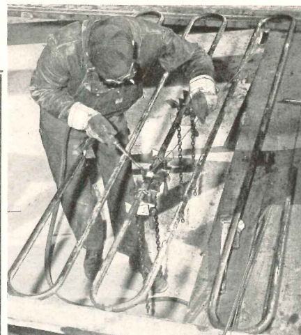
Buttweld steel pipe, designed for ease of fabrication for radiant heating, is being used in Ohio State's new medical center
