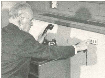
Valuable working time can be saved by conveniently-located switches in the General Electric remote control wiring system.
