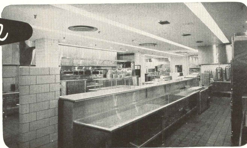
Kitchen of Terrace Plaza Hotel, Cincinnati; Skidmore, Owings and Merrill, Architects
