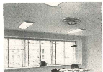
VENTURI-FLO CEILING OUTLET IN OFFICE
