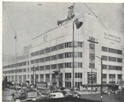
Newspaper plant and radio station nearing completion in Louisville is really two buildings, but gives appearance of one
