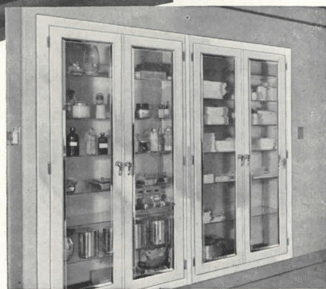
Recessed supply cabinet in septic operating room
