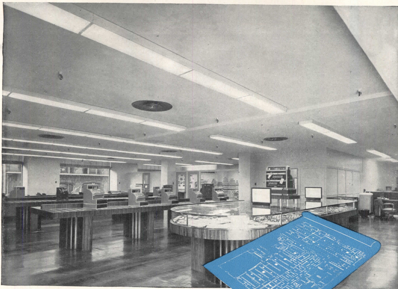
Showroom of the National Cash Register Company, Rockefeller Center, New York City. L-I-N-O-L-I-T-E Series 11, two 40 watt lamps, louver shielded fixtures (11-248L) were used to obtain 35 foot-candles maintained.
