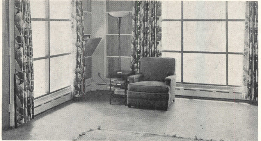
Fig. 4: typical installation of radiant baseboard
