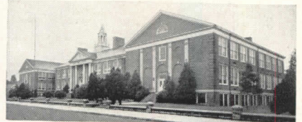
Salem High School, Salem, N. J. Built 1912. Wings added 1927. Steam heat distribution modernized 1946 with Webster "Controlled-by-the-Weather" Moderator System. Modernization Heating Contractor—William J. Kelly, Inc., Camden, N. J.
