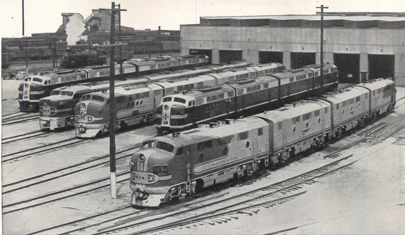
● Sidewalls of this Diesel engine house of the Santa Fe Railway at Barstow, Cal., were constructed of K&M "Century" Asbestos Corrugated.
