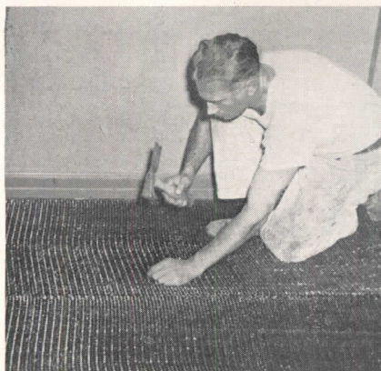
Steps in installing oxychloride cement floor over wood subflooring. Left, metal lath is nailed down over waterproof paper (neither is required on concrete subflooring which is broom finished). Center, the plastic mix is leveled off about \frac{1}{2} in. thick. Right, after the cement has been troweled and allowed to set, the finished floor is sanded
