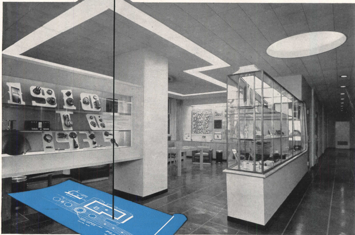
A modern showroom, illuminated by L-I-N-O-L-I-T-E Series 15 Troffers with four 40W lamps and louver bottoms, and custom built circular cove lighting.
