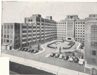
Delaware Hospital, Wilmington, Delaware. Heated by 6-zone Webster Moderator System of Steam Heating. Completed in 1942. Unit No. 1, center, occupied in 1940. Architects: Massena & duPont, Wilmington. Consulting Engineers Jaros, Baum & Bolles, New York. General Contractor: Turner Construction Co., Philadelphia. Heating Contractor: Benjamin F. Shaw Co., Wilmington.
