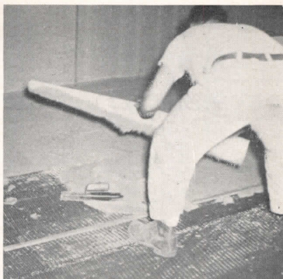
Steps in installing oxychloride cement floor over wood subflooring. Left, metal lath is nailed down over waterproof paper (neither is required on concrete subflooring which is broom finished). Center, the plastic mix is leveled off about \frac{1}{2} in. thick. Right, after the cement has been troweled and allowed to set, the finished floor is sanded
