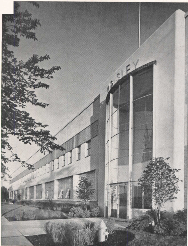
Ground to roof facade of Allen B. Wrisley Company, Chicago, has continuous panels of Insulux Prismatic Glass Block. Three face patterns and approximately 4500 glass blocks provide the ultimate in daylighting this modern and progressive plant. Architects: Fugard, Burt and Wilkinson, Chicago Ill.
