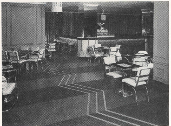
Resilient flooring material gives the architect many opportunities to carry out the theme of the interior in the floor design. Here the military motif of the room's decorative scheme is picked up in the stripe and chevron design of the floor. Two colors of jaspé linoleum form the stripes, while plain linoleum was used in the rambling chevron design.
