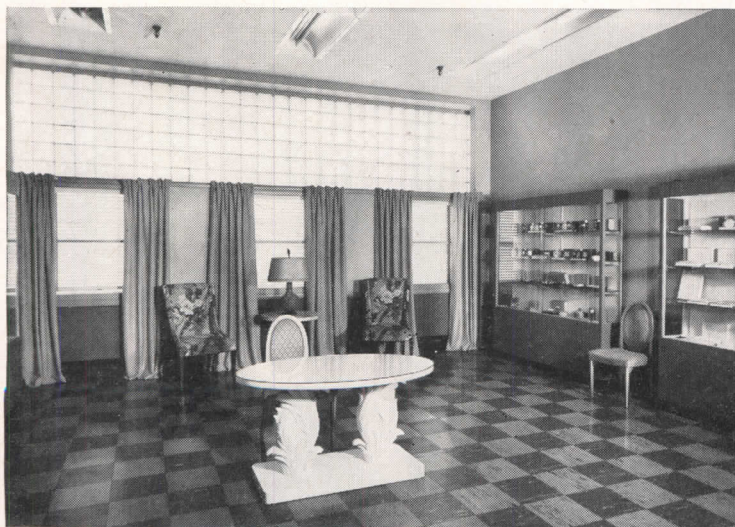
Insulux Prismatic Glass Block turns light to ceiling for re-direction into this second-floor display room. Drapes over windows can be entirely drawn without loss of daylight in room. Same type panels give fine working light in factory areas.
