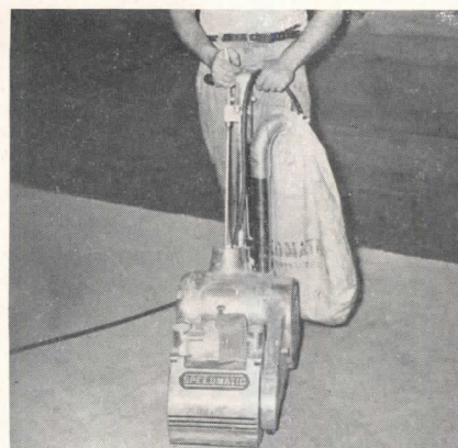
Steps in installing oxychloride cement floor over wood subflooring. Left, metal lath is nailed down over waterproof paper (neither is required on concrete subflooring which is broom finished). Center, the plastic mix is leveled off about \frac{1}{2} in. thick. Right, after the cement has been troweled and allowed to set, the finished floor is sanded
