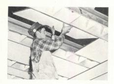
Panels of acoustical Fiberglas fit between light troffers to form a suspended ceiling
