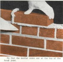
All head joints in both face brick and back-up work should be completely filled with mortar. One good method for doing this is to throw plenty of mortar on the end of the brick to be placed. (This should be done in such a way that the mortar is scraped off the trowel by the bottom edge of the end of the brick.) Then push the brick into place so that the mortar oozes out at the top of the head joint.
