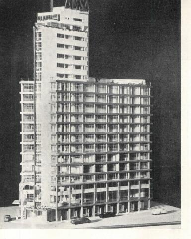
Model of the A.M.S.A. Insurance Building, Mexico City, Enrique del Moral and Mario Pani, architects. The reinforced concrete skeleton is exposed above the third floor where the glass walls are behind the columns. On the second and third floors, the glass wall extends in front of the columns
