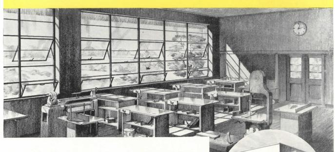
This school training shop exemplifies the versatility of Standard Fencraft Windows. It calls for abundant daylight . . . plenty of ventilation and good control of it. The use of medium size panes is recommended for easy, low-cost glass replacement. Sill vents that discourage leaning out of windows are desirable.
