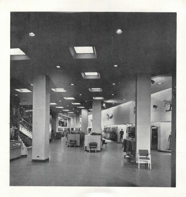
Photo above is general view immediately after passing outside pylon with show case (see photo, page 91, lower right), and through the clear-glass main-entrance doors. To secure proportions of height necessary for this sweep of nearly 200 ft., the architects used slide-rule ingenuity to minute inch fractions in reducing the depth of their dropped plaster ceiling to absolute minimum. Not only does it conceal air conditioning ducts and conduit for the store's incandescent "pots" and fluorescent
