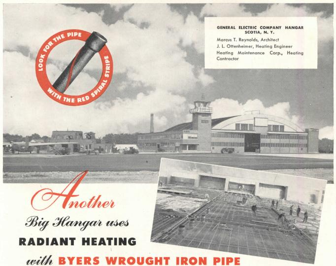
With a floor area 168'8" square, a roof 45' above grade at its high point and 17' at the eaves, and large, frequently-opened access doors, this hangar, like all such structures, presented a difficult heating problem. The designers solved it with radiant heating, which has been successfully used in a number of similar applications.
