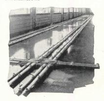
For wiring flexibility in concrete office buildings, plants, hospitals, and for other construction jobs where provisions must be made for varying wiring needs, look into the advantages of Fiberduct underfloor raceways. These nonmetallic, corrosionproof ducts permit installation of new outlets anywhere in the duct at any time. Buildings equipped with Fiberduct stay electrically young. See us for detailed information
