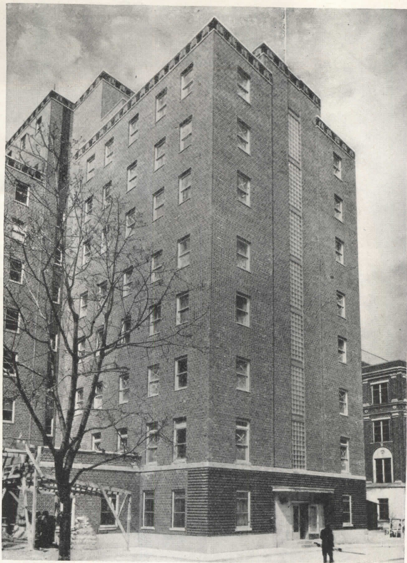
Eight stories in height, this 50 bed, solarium-equipped addition to the New Rochelle Hospital, New Rochelle, N. Y., used 32½ tons of Bethlehem Open-Web Joists. Contractor: Turner Construction Co., New York. Architects: Shreve, Lamb & Harmon Associates, New York.
