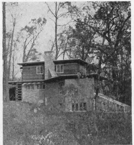
The living-room end of the wing-nut plan utilizes natural contours to put greenhouse (on south wall) at basement level, and to give maid's room, bath full window height
