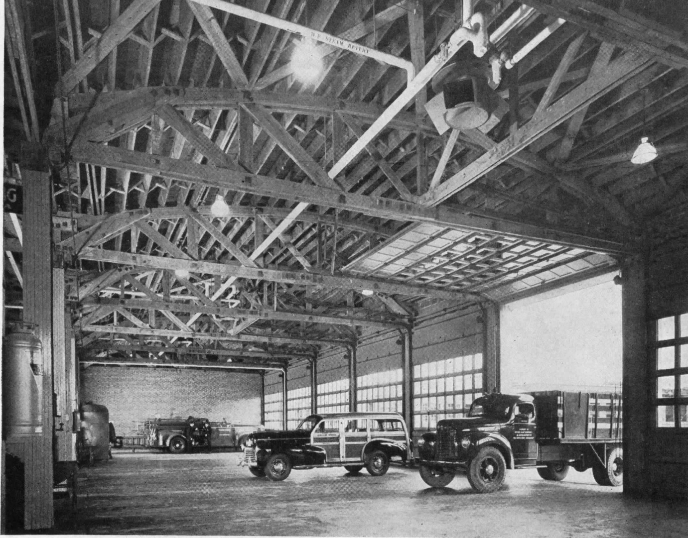
The truck garage building was built with lumber from the huge movable forms used for concrete work in the main manufacturing building. Here columns, roof trusses and roof itself are of wood, most of it taken from the concrete forms
