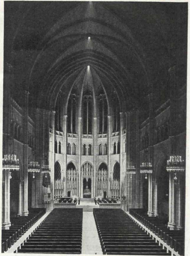
Figure 1, left, shows the type of "general" lighting used in New York City's Riverside Church. Figure 2, right, with "specific" lighting added
