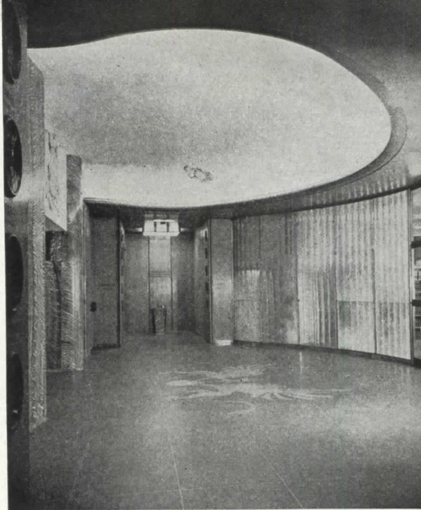
Fifth floor lobby (above) has cast glass screen partitioning in a blue-green tone, clear glass panels in doors to the law library. Floor is of black terrazzo
