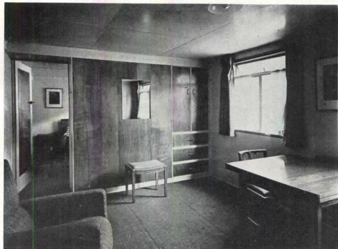
One wall of well-proportioned living room is cupboard unit backed on bedroom side by wardrobe, drawers and linen shelves
