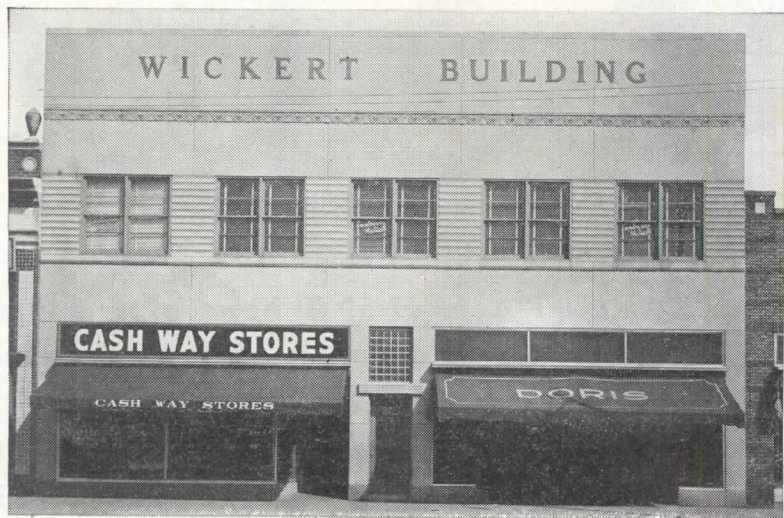
ARCHITECTURAL CONCRETE SLABS applied over old brick finish on the Wickert Building, Escanaba, Mich. The facing is buff; base course is green; and the monolithically cast raised letters are in green vitreous aggregate. The matrix is Atlas White cement. Architects: Hubert & Gjelsteen, Menominee, Mich.; Contractor: Mike Rettman, Bark River, Mich.; Slabs by Badger Concrete Co., Oshkosh, Wis.
