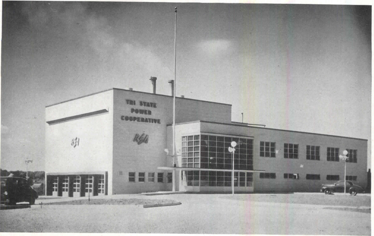
The Dairyland (formerly Tri-State) Power Cooperative, one of the prewar REA plants. Roland A. Wank, architect; A. Y. Taylor & Co., engineers
