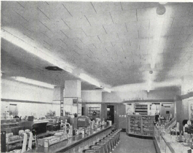
Drug store lighting by means of fluorescent fixtures with translucent louvers transverse to the long axis
