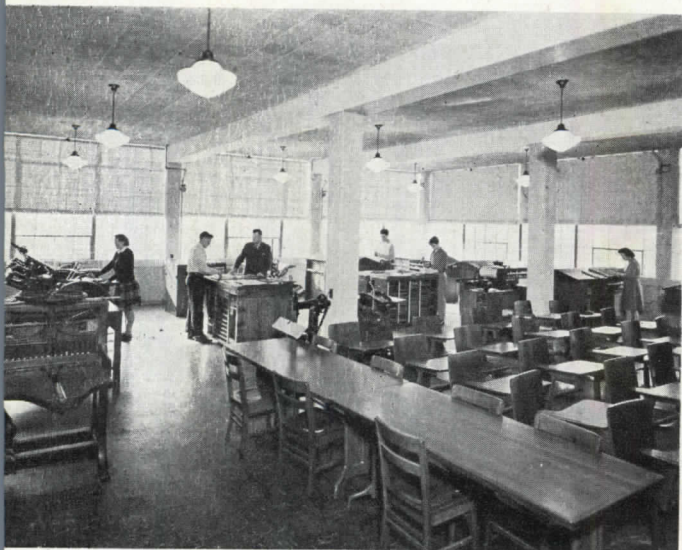
Printing shop has second floor corner location; note the continuous windows around type-setting tables and presses
