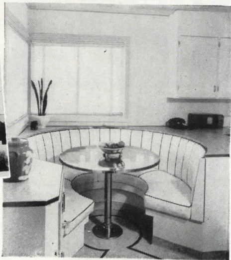
Lorenzo Mansfield designed this smart circular breakfast room, built of Douglas Fir Plywood. A similar installation rejuvenates any kitchen.
