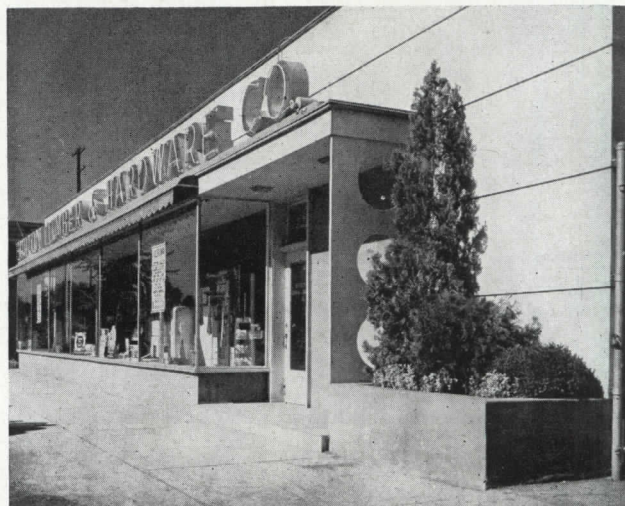
An effective remodeled store front in Salt Lake City done in simple materials by Lowell Parrish, architect.
