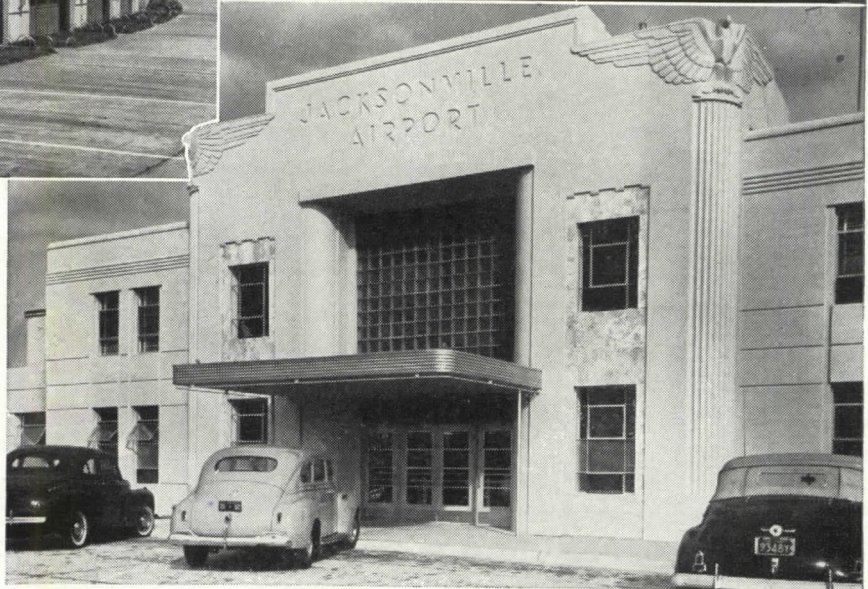
Below—Decorative details on administration building at Jacksonville, Fla., Municipal Airport are an integral part of the architectural concrete structure designed by Jefferson D. Powell, Jacksonville architect.
