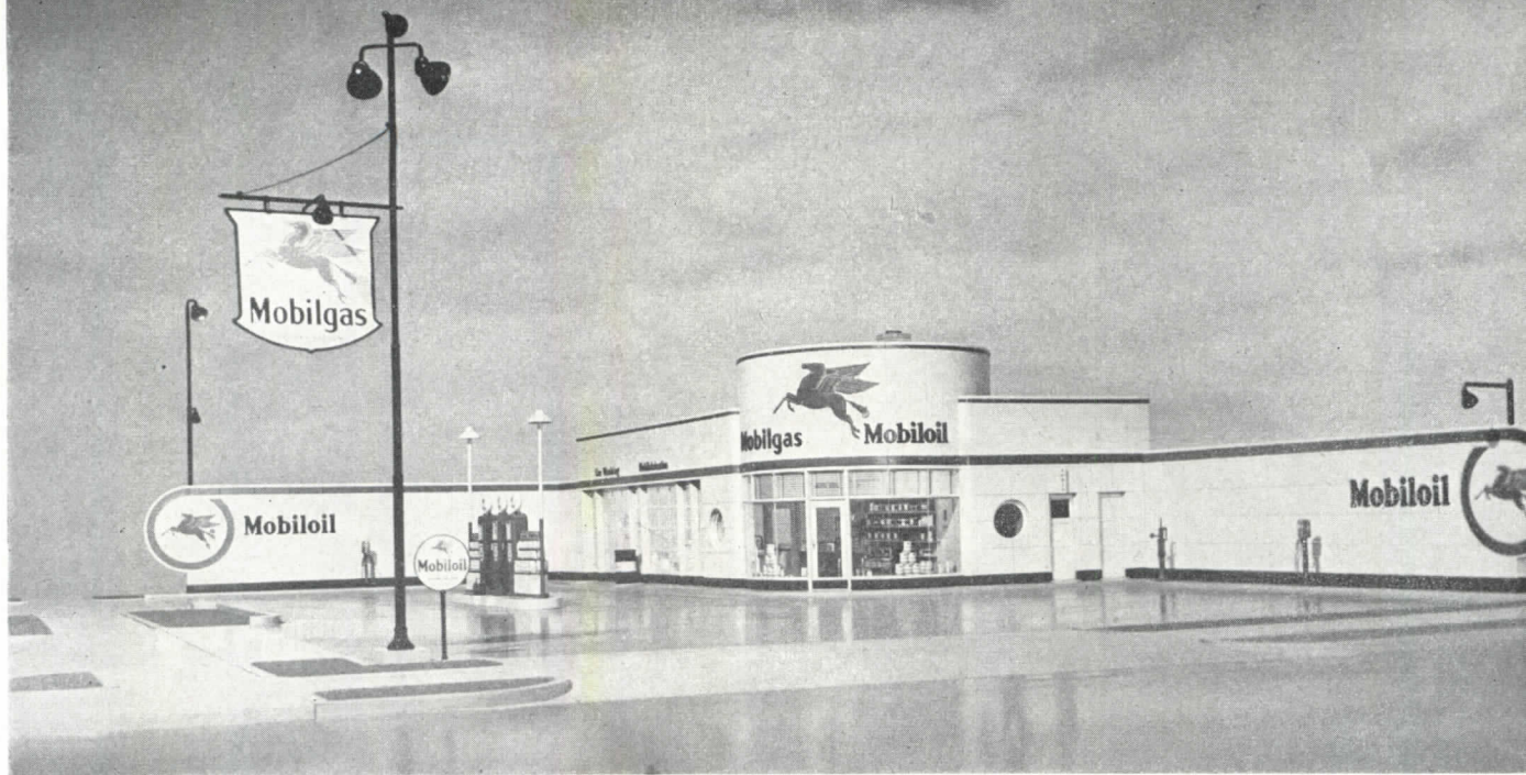
Advanced station model in current use: Frederick Frost, architect. The "drum" shape is a trademark. Porcelain enamel finish, standardized elements, efficient arrangement, good screening
