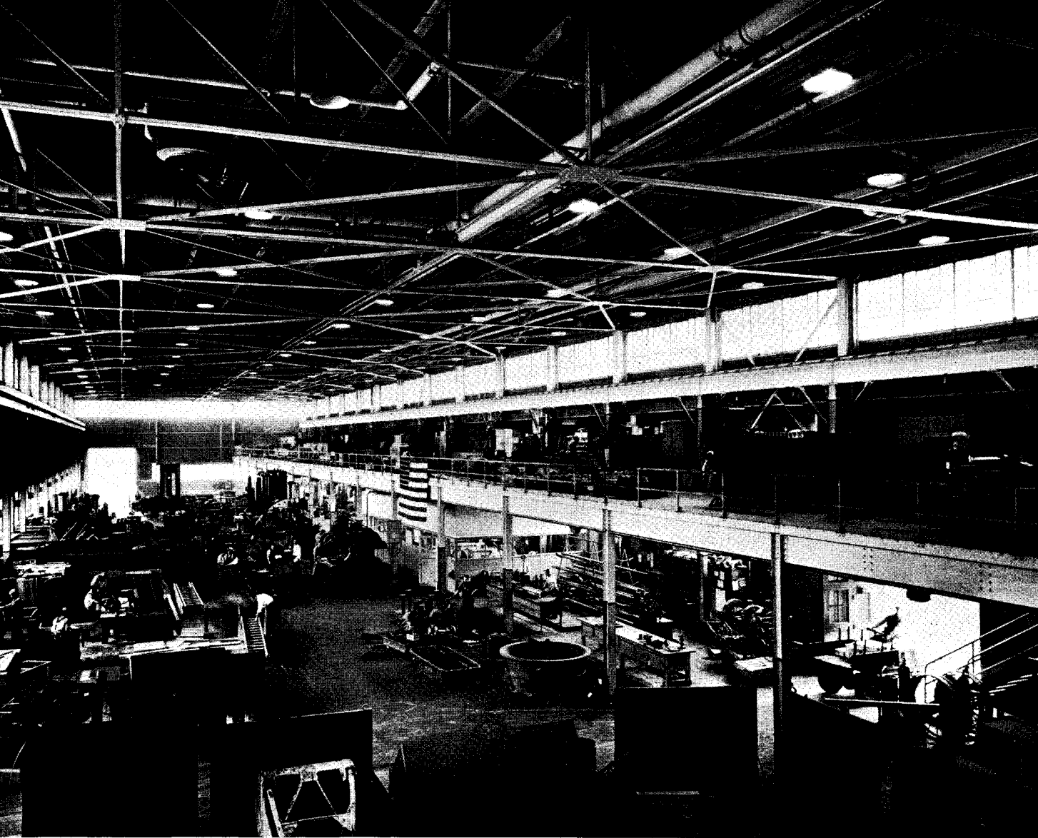
One of the smaller structures in the main group, the maintenance building measures 700 by 76 ft.
