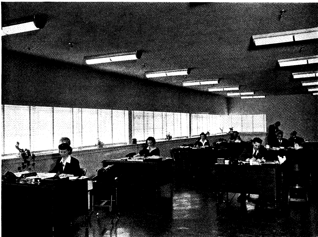
General office space has complete air conditioning, acoustic ceilings, asphalt tile floors, fluorescent lighting
