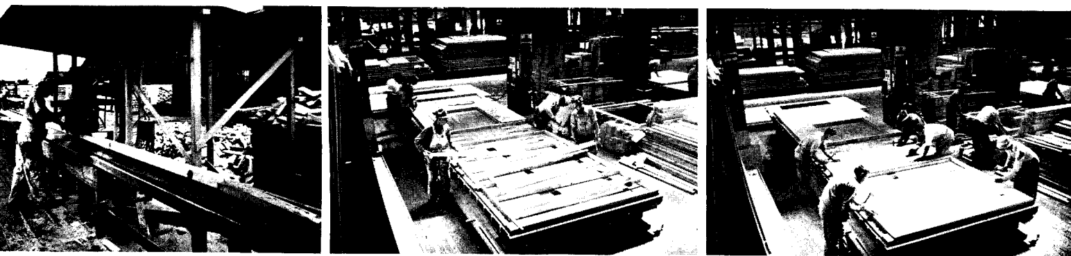
First of the really large-scale site prefabrication projects of Homasote houses done by Barrett & Hilp, this one the now-famous Vallejo, Cal.,
