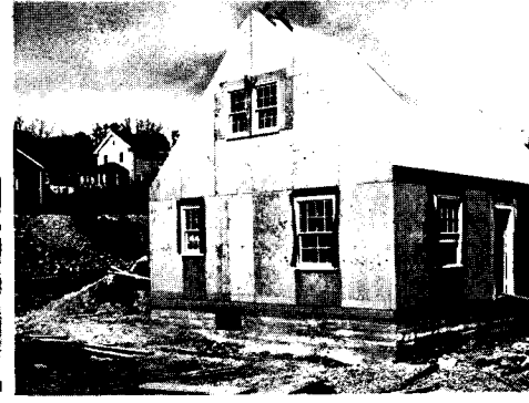
here they demonstrate that a few men can erect the structure in a few hours, in this case starting at 8 A. M., and finishing at 3:55 P. M.
