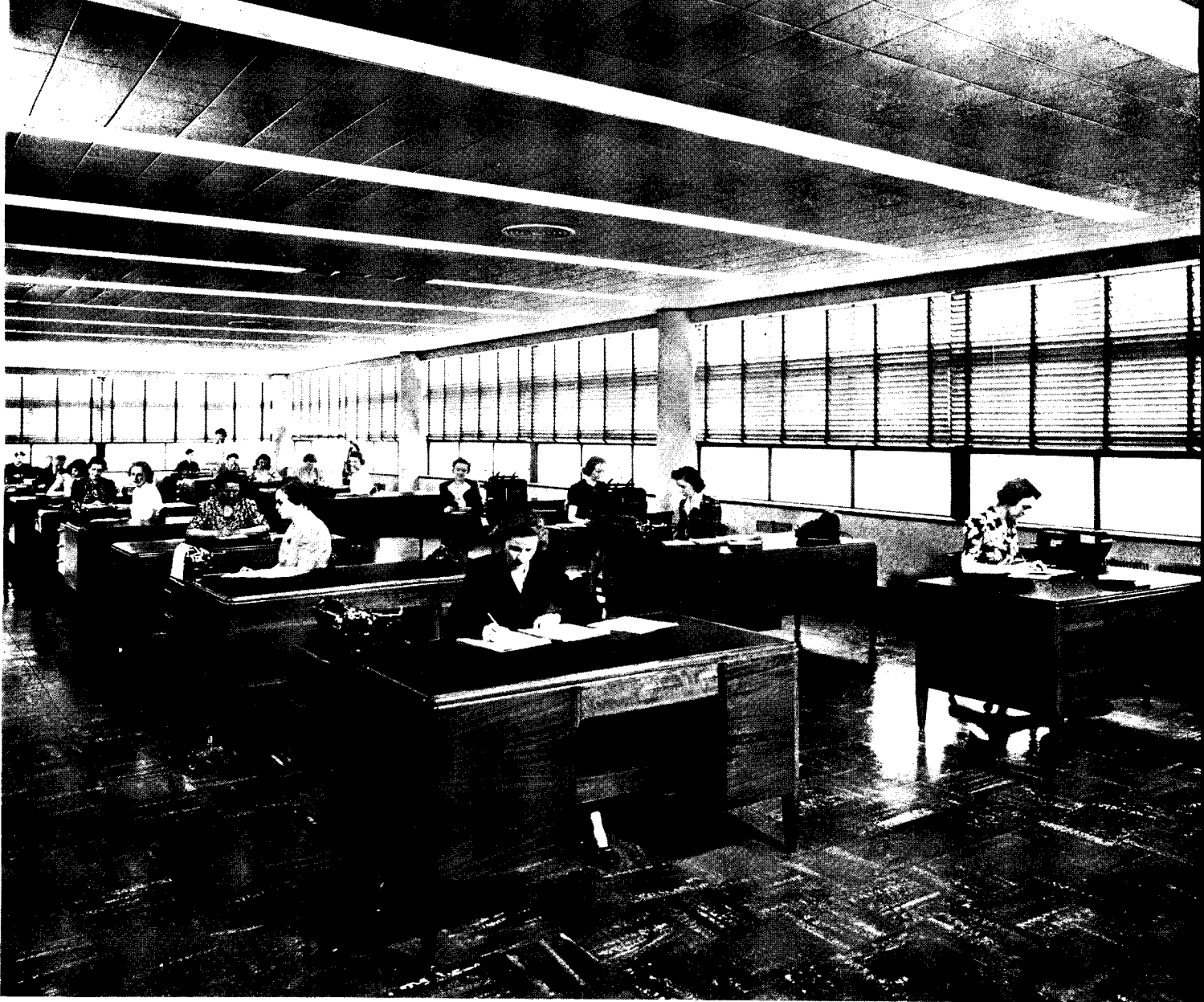
General office space on the third floor has full windows, fluorescent lighting, acoustical ceiling, asphalt tile floor, air conditioning
