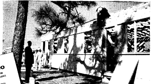
Cemesto construction is sturdy and economical. Houses are finished at the rate of 20 a day.
