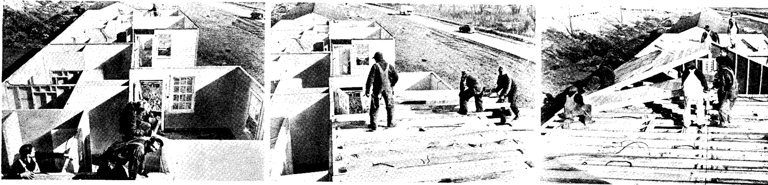
panels being built in a plant at North Tonawanda, N. Y., trucked to box cars, and being assembled in Dayton, Ohio, in a war housing project
