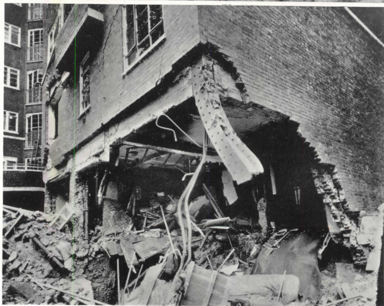
1. Steel-framed structures have the ability to withstand severe punishment from bombing without disintegrating as is the case with plain masonry structures.
