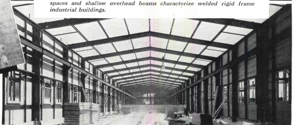
Continuity of members at their intersections permits a reduction in their size and provides more lateral stability. Welding facilitates the making of such connections.
