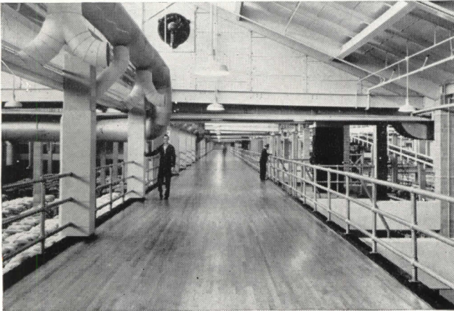
National Biscuit Company, Atlanta Bakery floored with Northern Hard Maple. Photo, courtesy G. H. Tennant Co., Minn. Louis Wirsching, New York City, Architect.
