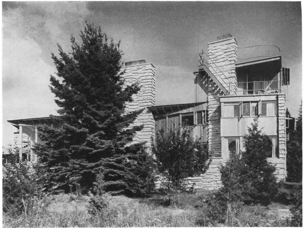
At right. The west elevation showing bedroom wing with recreation room below. The exterior stairway leads from the studio terrace to the high sun deck with its wide view.
