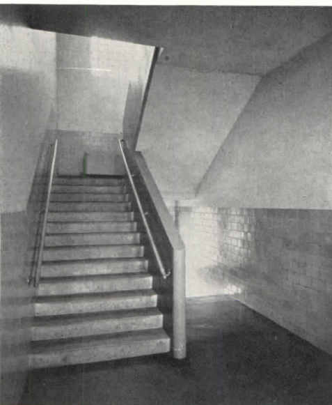
CONCRETE stair and balustrade: low maintenance, great safety, permanence. Ocean View School, Norfolk, Va.; V. A. Moore and Associates, Architects
