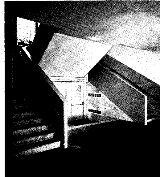
ENTRANCE, exterior and interior; note the so concrete stair rail and the well-lighted landing
