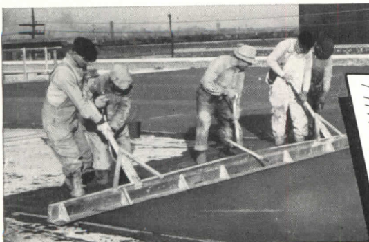
★★★ CHANUTE FIELD, the nation's foremost air training center. ZONOLITE CONCRETE used for insulating roof fill over almost four acres of concrete roof deck—and for all saddles and cant strips. Photo courtesy of U. S. Army Air Corps. ★★★
