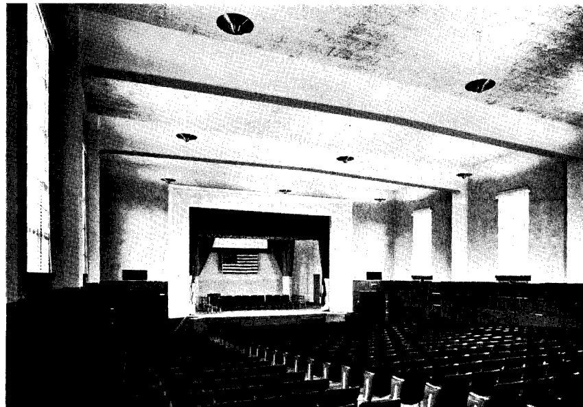
AUDITORIUM has exposed, rigid, concrete framing
