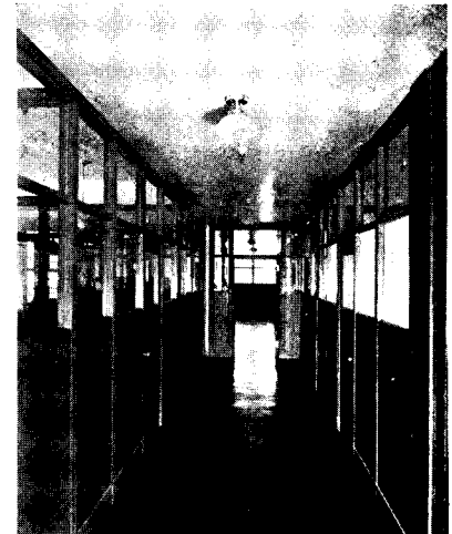
Office partitions are metal and glass
