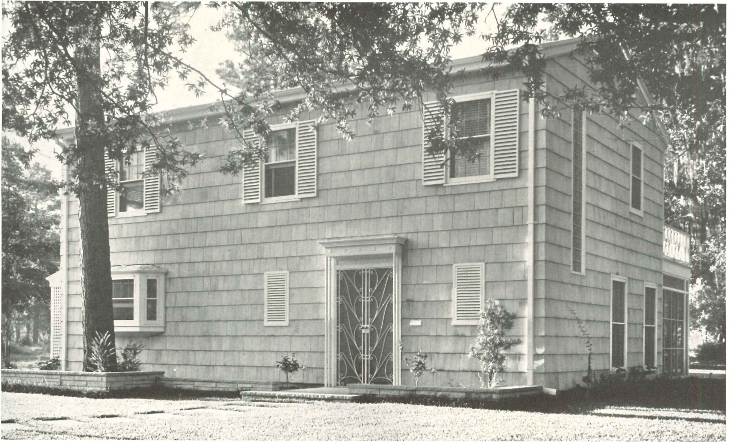
MR. MACKIE'S own house. Economy of construction and low-maintenance considerations are as noteworthy as the efficient organization of plan. The house is built on a concrete slab. Shingles are stained light gray; trim is white; the built-up fireproof roof has a white limestone topping. All rooms have cross ventilation. The generous screened porch at the rear, equipped with a barbecue fireplace, is the center of summer living.
