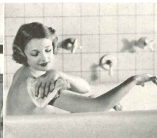
Low cost, year around domestic hot water
