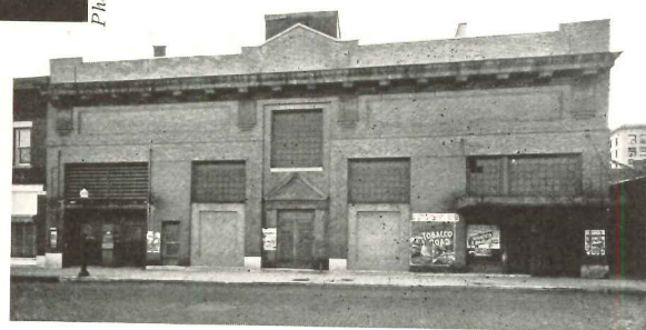
Old theater building before remodeling
