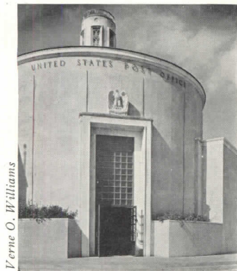
Fig. 11. Concrete walls, formed against plywood, were used in the Miami Beach, Fla., post office. Howard Lovewell Cheney, Consulting Architect for Procurement Division, Treasury Department.
