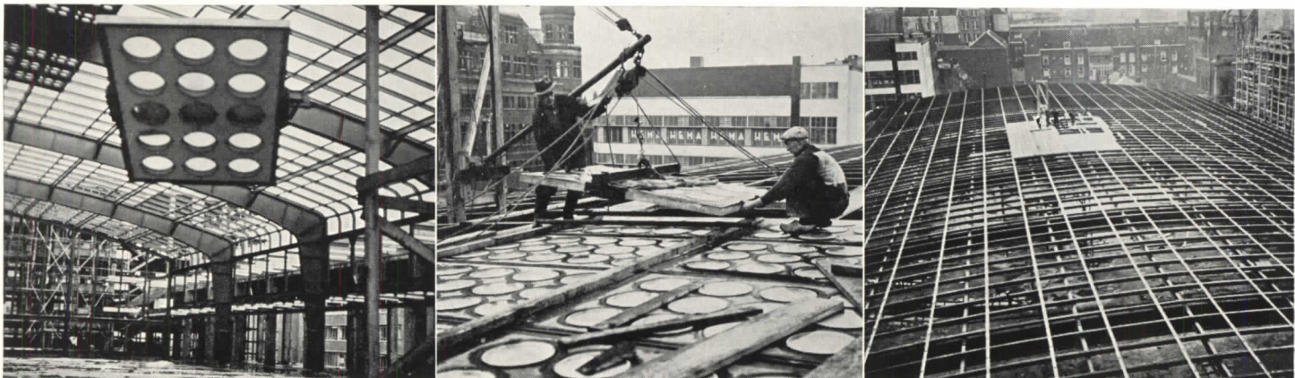
Glass-crete units are raised to roof . . . projecting ribs fit into U-shaped purlins . . . which run between welded arched girders.
