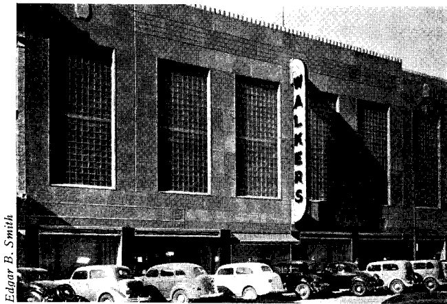
Fig. 21. The new exterior of Walker Department Store, Wichita, Kan., is of 1 3/4-in. precast slabs, up to 4 by 6 in. in size, faced with dark green crushed marble exposed by brushing. Lorentz Schmidt, Architect. At left, exterior before remodeling.
