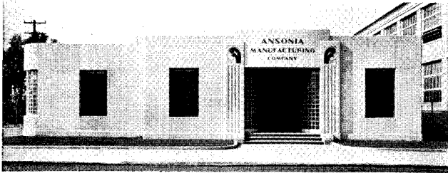
Fig. 20. Large, quartz-faced slabs, 2 in. thick, backed up with concrete masonry units reduce joints to a minimum on this building of Ansonia Manufacturing Co., Ansonia, Conn. Brown and Von Beren, Inc., Architects.
