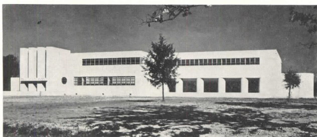
Fig. 12. Notable success in the use of concrete in the Columbia, Miss., high school. N. W. Overstreet and A. H. Town, Architects.
