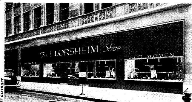
Fig. 22. Highly polished slabs, 2 in. thick, made with a mixture of blue and green granite chips, were used in remodeling this store in New York City.
