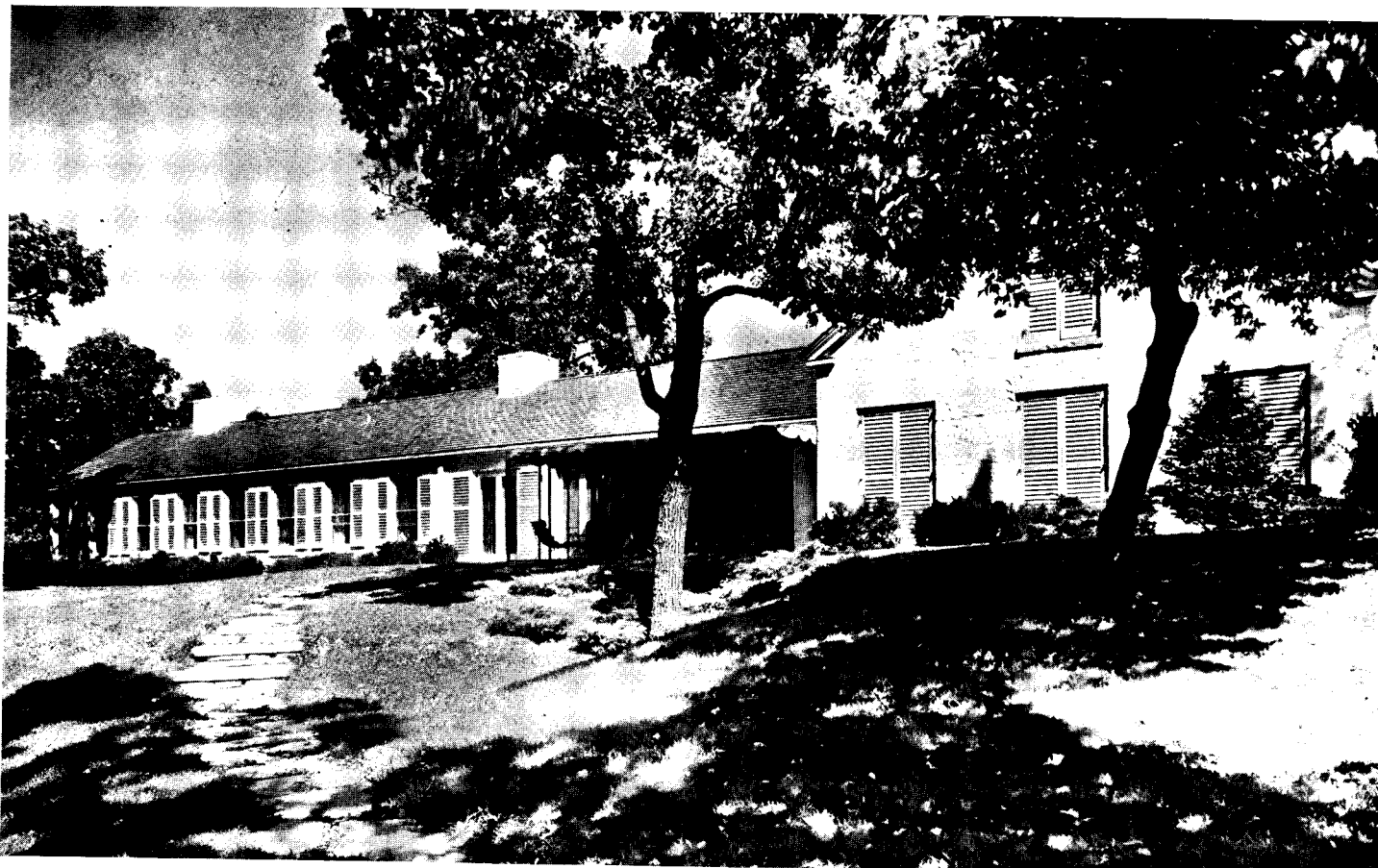
The rear side of the house is more open and informal than the front; the terrace opens off living and dining rooms
