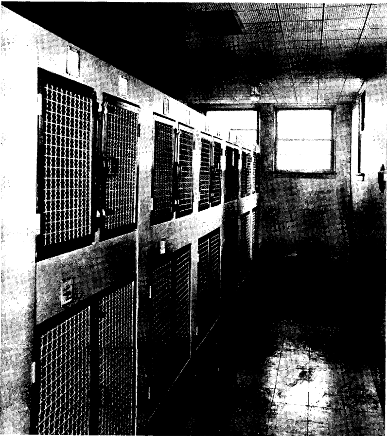
Kennels for sick animals: A cane-fiber material (Acousti-Celotex) applied to the ceiling deadens the din of barking.
