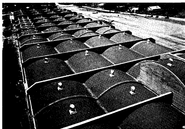
Fig. 7. Longitudinal barrel shells make up the roof of the Armstrong Tire and Rubber Co. factory, Natchez, Miss. Within the building, bays are 40 ft. wide and columns are 50 ft. apart in the longitudinal direction. J. T. Canizaro, Architect; Roberts and Schaefer Co., Engineers.
