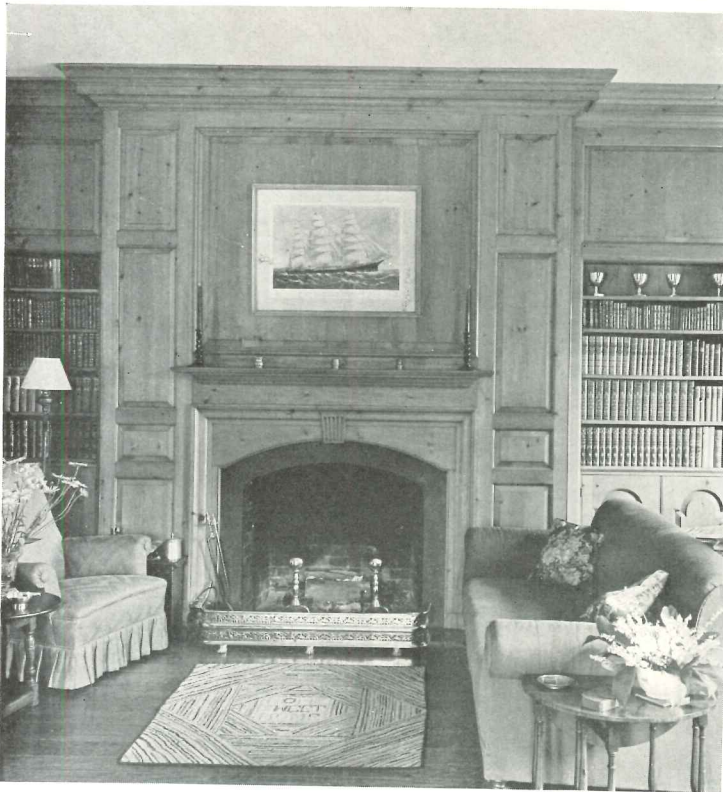
The dining room mantel, shown at the top, is an original from Williamsburg and has been incorporated in the wall treatment. Paneling and niches are new. The library mantel, shown below, is of pine; mantel, paneling, and bookshelves, designed for the house, are detailed at the right.
