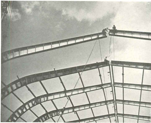
Aviation Building's solid-web arch trusses are swung into place.
