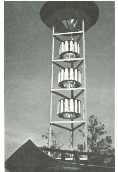
Zeon lighting on Information Booth. Fair Board of Design, architects.
