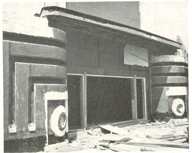
Stucco on metal lath, Transportation Building. James Gamble Rogers, architect.
