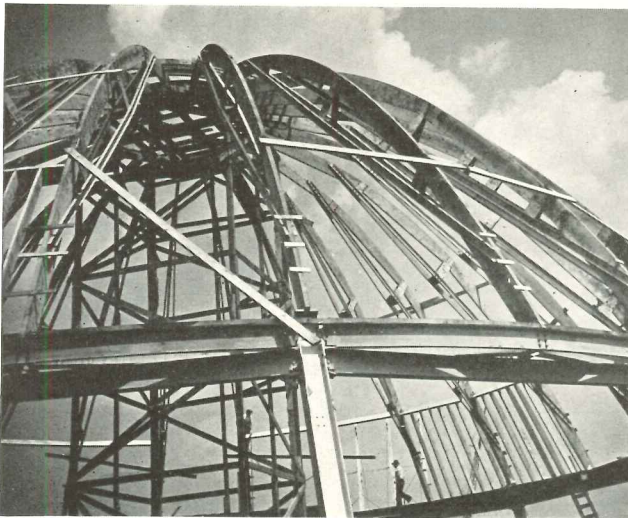
Wood templates in place on dome of Distilled Spirits Building, timber studding follows.
