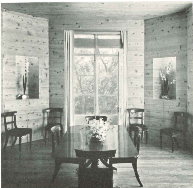
Above, interior of living-room; below, dining-room. All same walls are finished with knotty red cedar board-and-batten. Wood studs and plates are secured to adobe walls with bent lengths of barbed wire embedded in mortar joints and nailed to framing.
