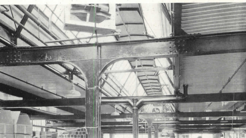
Simplified assembly using welded "Columbeam Construction" bolted to running members
