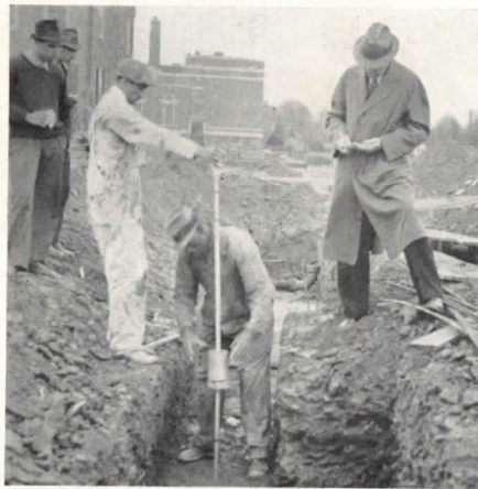
Method of testing soil with "Drop-Penetration Rod". Load-bearing values are determined by noting the number of times a sliding weight must be successively dropped against the collar to drive rod each foot.
