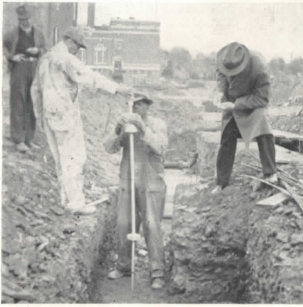
Method of testing soil with "Drop-Penetration Rod". Load-bearing values are determined by noting the number of times a sliding weight must be successively dropped against the collar to drive rod each foot.
