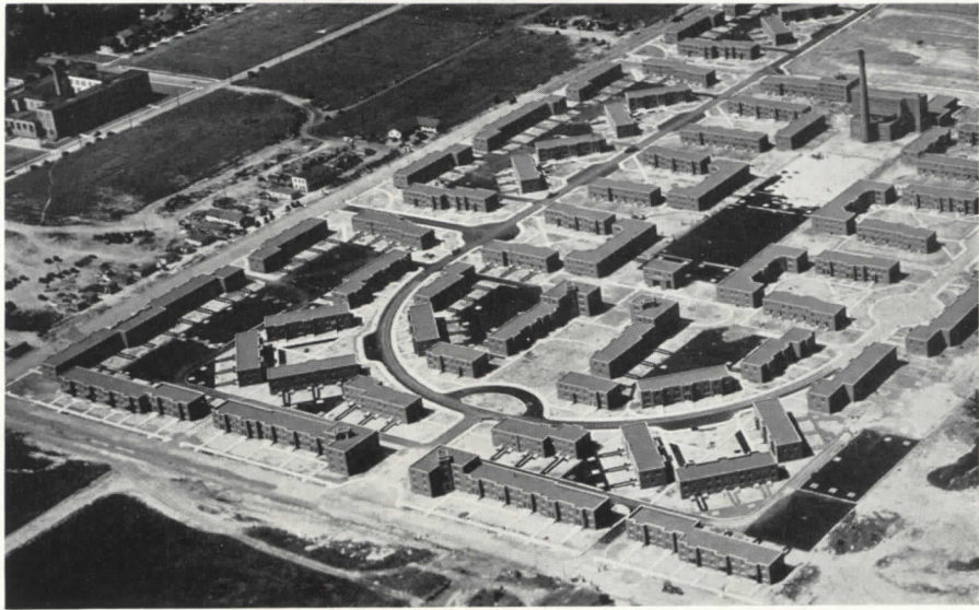
Site development, government housing in Austin, Texas
