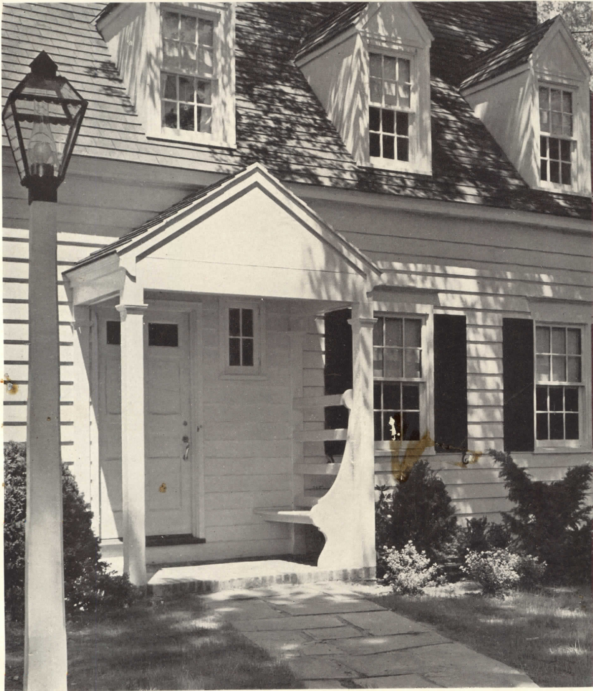
Detail of Front Entrance from the South
