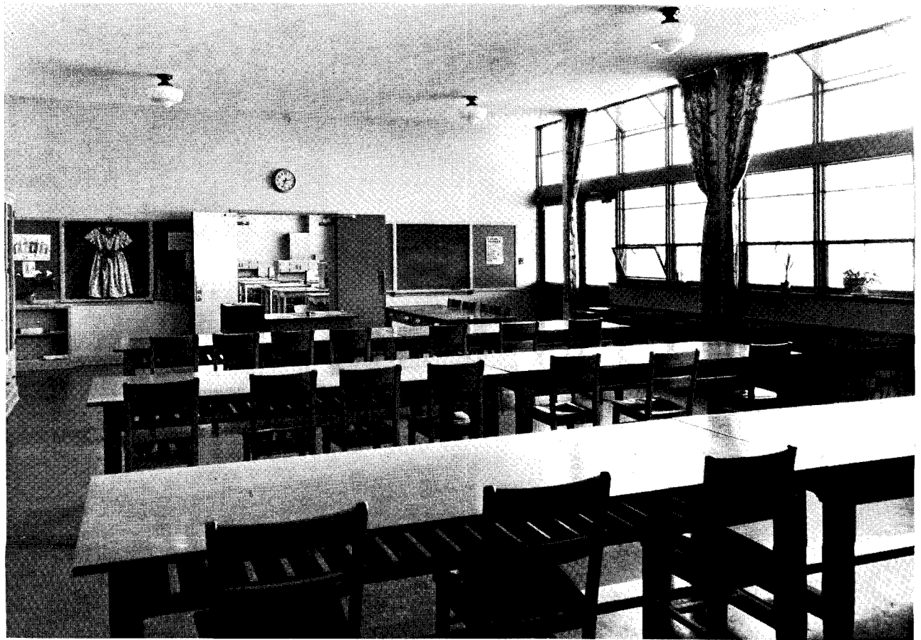
Sewing Room, Practical Arts Building. Note uniformity of natural lighting above and below colonnade roof.
