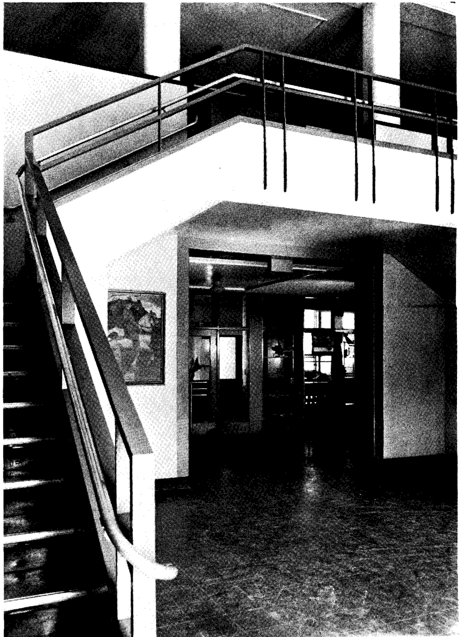
Main Stair Hall, Academic Building. Stairs have cork tile treads, aluminum nosing. Note plate glass on both sides of trophy display case.
