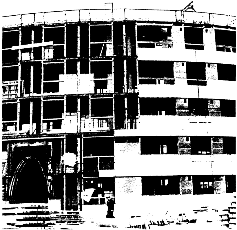
Stage 2: Concrete slabs in place
