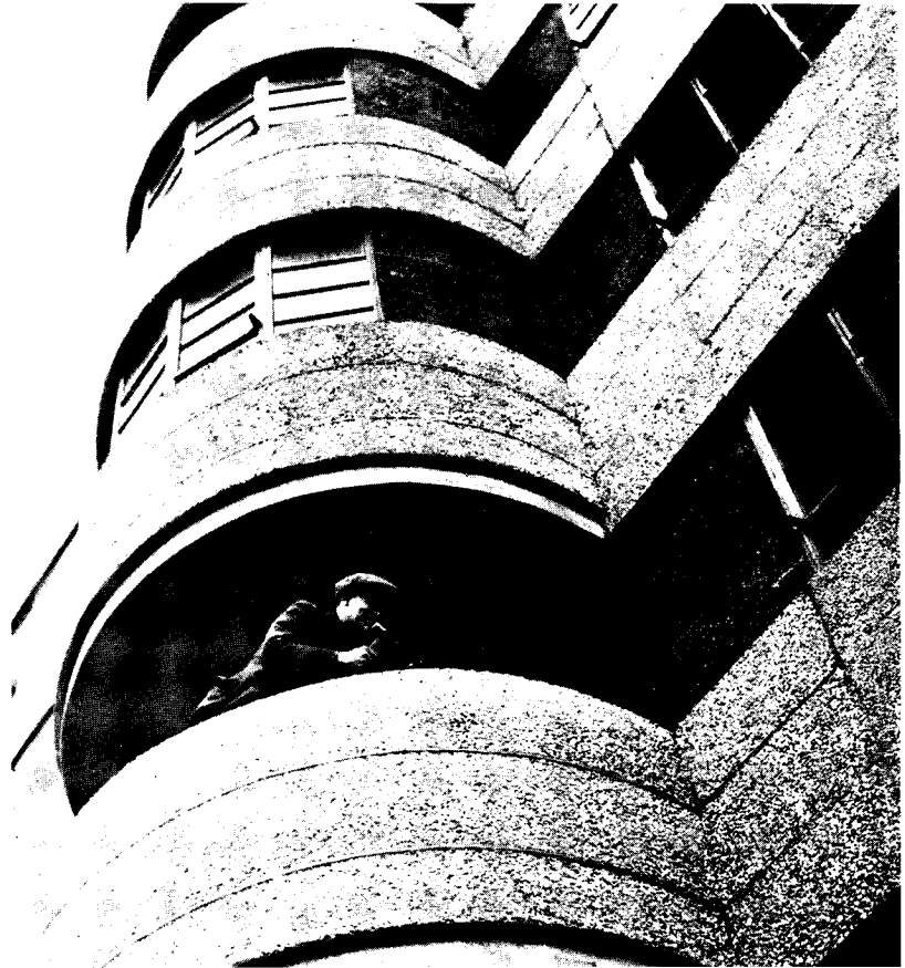
Stage 3: Finishing the exterior
