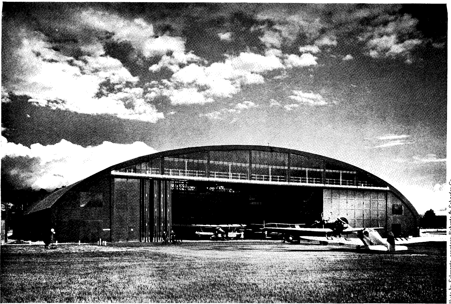
Airplane Hangar, Germany. Construction is monolithic concrete, Z-D system. Concrete shell is 4\frac{3}{4} in. thick. Span is 165 ft.
