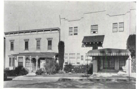
Building before alteration
