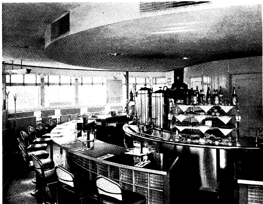
Equipment for counter service is compactly arranged and connected by swinging doors with the kitchen. Table service is handled through the door at the upper right of the picture. Floors: black terrazzo with aluminum strips. Walls: cream-colored Marlite on 2"x3" furring; surfaces between windows covered with flesh-tinted mirrors; wainscot, peach. Ceiling: acoustical plaster. Lighting fixtures: brushed aluminum.
