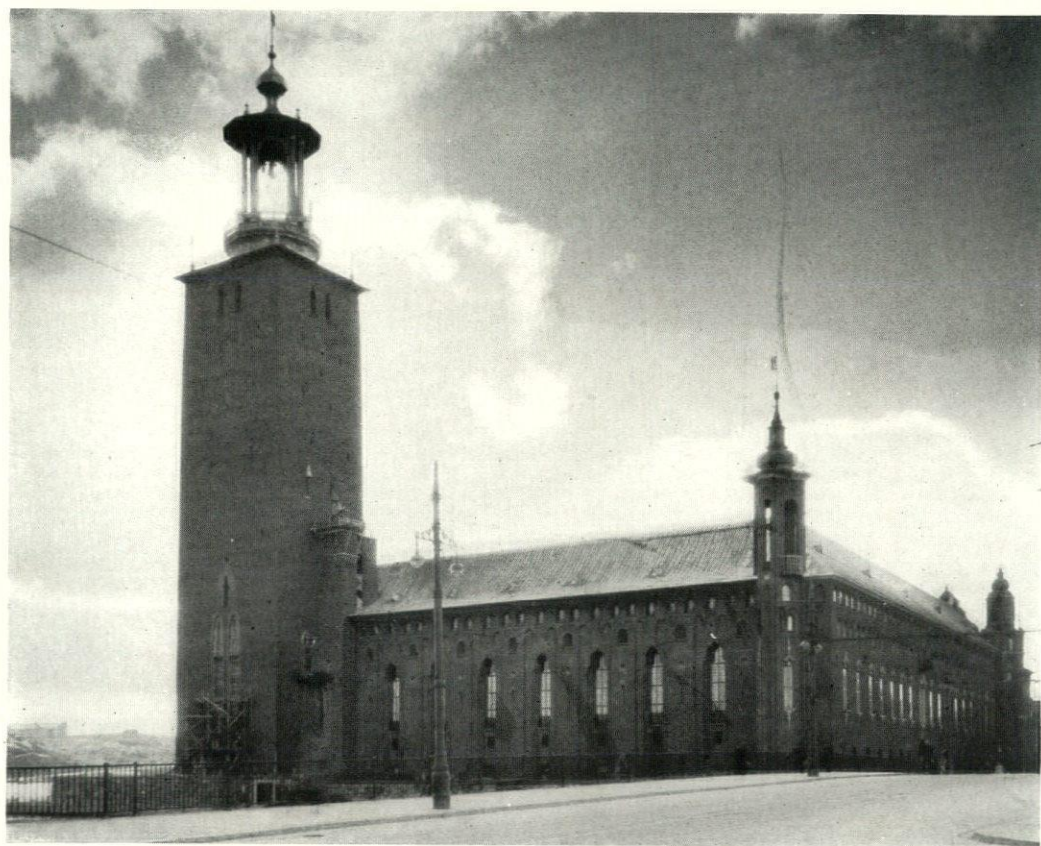
THE NEW CITY HALL, STOCKHOLM, SWEDEN Ragnar Östberg, Architect
