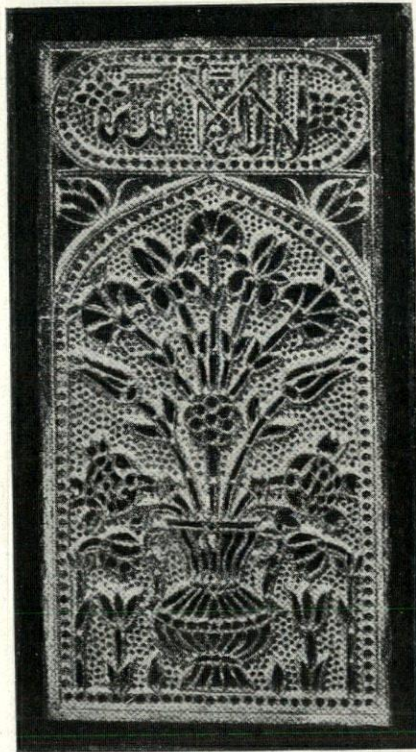
Kamariyyeh , or perforated plaster window with insets of colored glass, fourteenth century. (From the Manual d'Art Musulman , by Gaston Migeon)
