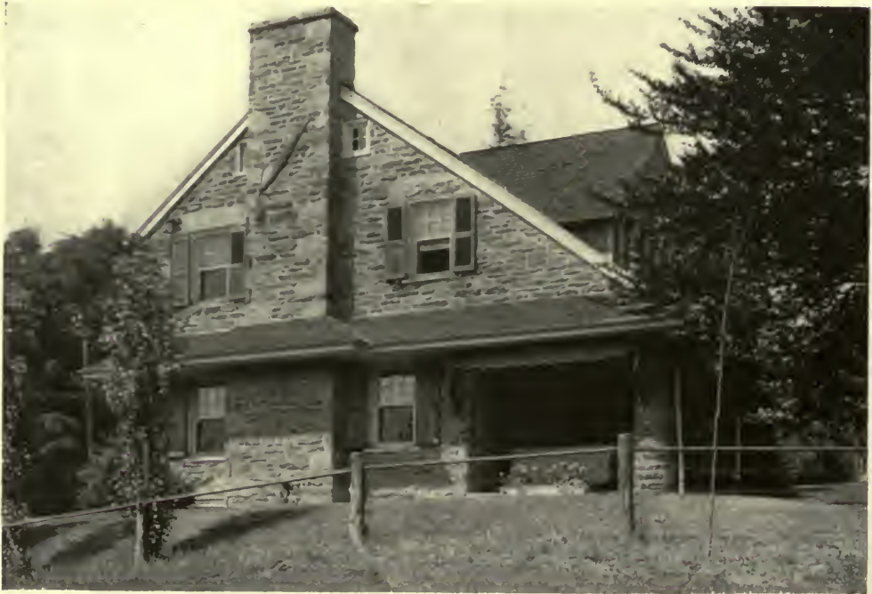
WEST FRONT—RESIDENCE OF MRS. JOSHUA L. SMITH, GERMANTOWN, PHILADELPHIA. Duhring, Okie & Ziegler, Architects.
