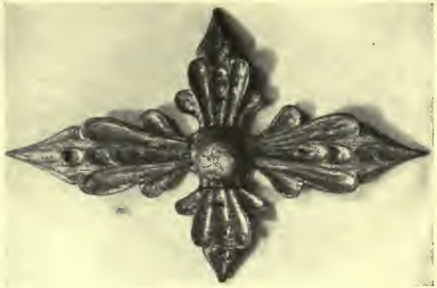
CORNICE ORNAMENT—MACLAY MANSION, HARRISBURG, PA.
