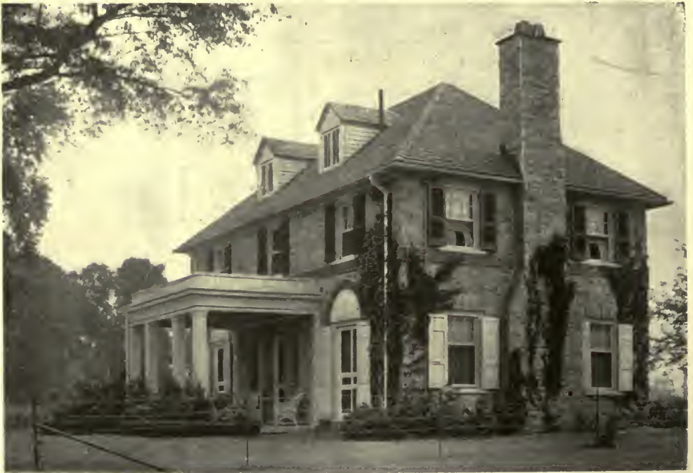
FRONT VIEW—HOUSE AT ARONIMINK, PA. Edward F. Hoffman, Jr., Architect.
