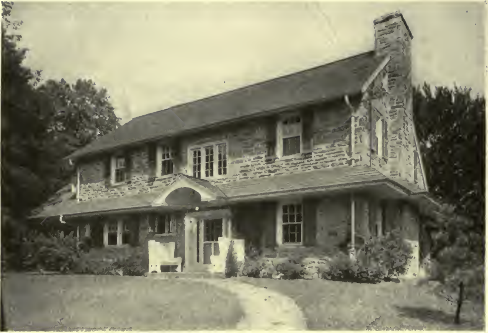
NORTH FRONT—RESIDENCE OF MRS. JOSHUA L. SMITH, GERMANTOWN, PHILADELPHIA. Duhring, Okie & Ziegler, Architects.
