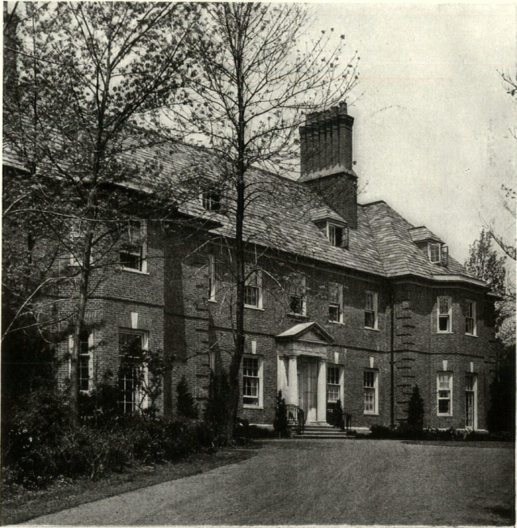
RESIDENCE AT HARTFORD, CONN. GOODWIN, BULLARD & WOOLSEY, ARCHITECTS.
