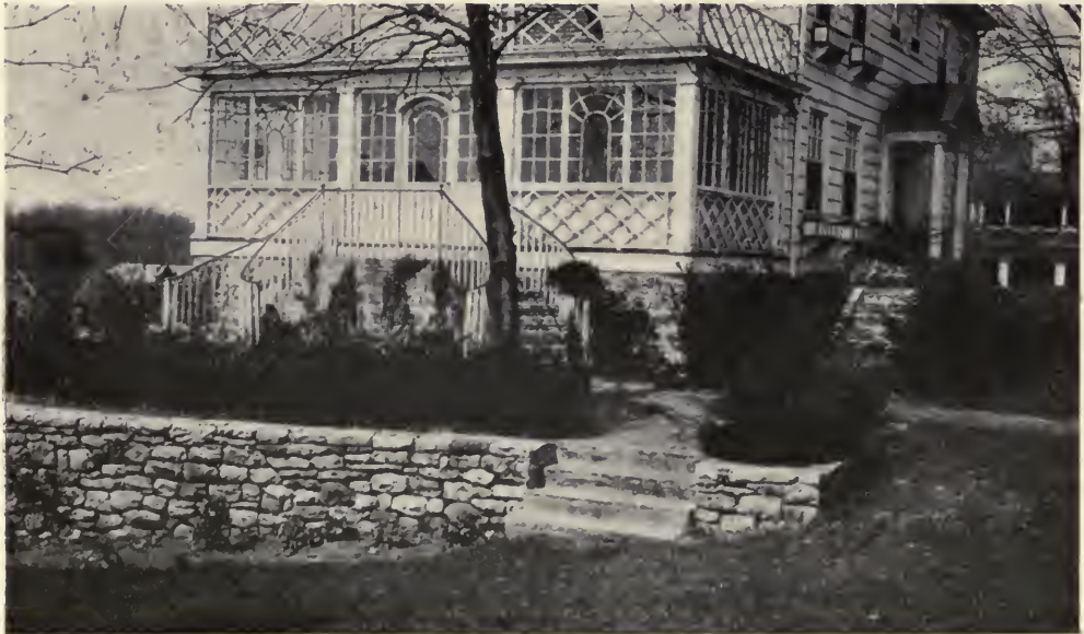
STEPS FROM GLAZED PORCH—RESIDENCE OF MRS. VINCENT B. THOMAS, HARTSDALE, N. Y. Frank Arnold Colby, Architect.
