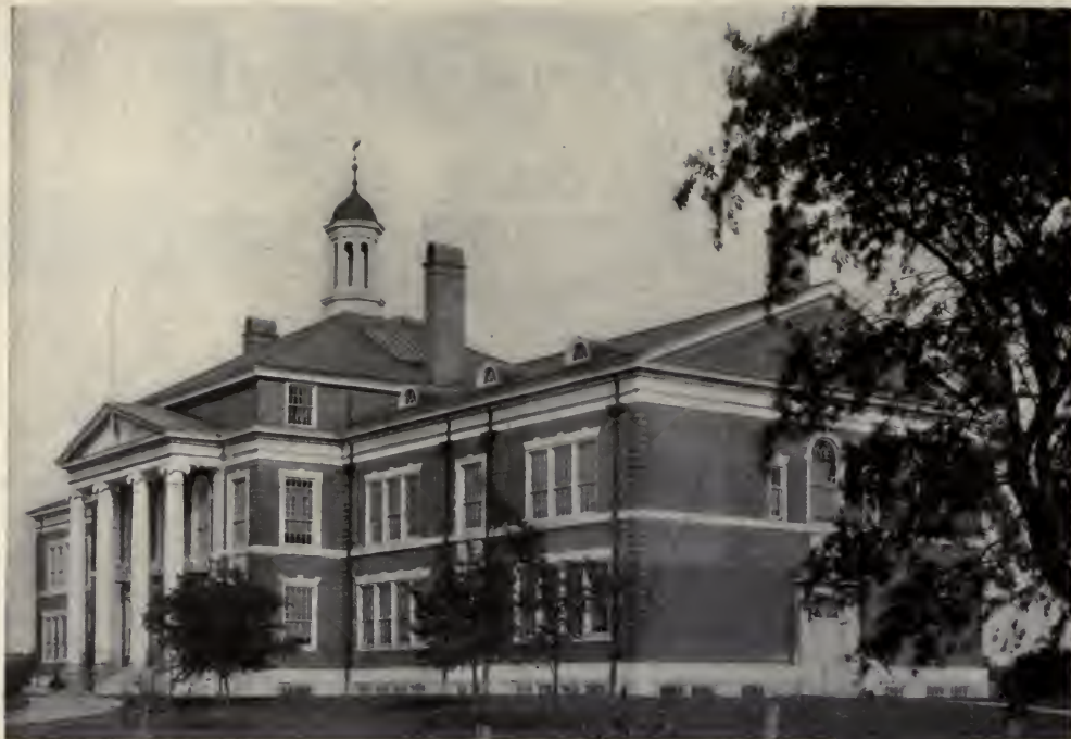
NORTH AND WEST FRONTS—HIGH SCHOOL, SOUTHAMPTON, L. I. William Lawrence Bottomley, Architect.
