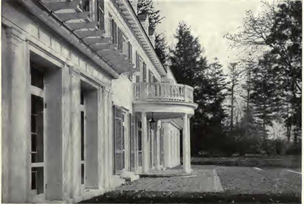
FIG. 62. RESIDENCE OF LEROY P. LEAS, ESQ., OVERBROOK, PHILADELPHIA, PA. Charles Barton Keen, Architect.
