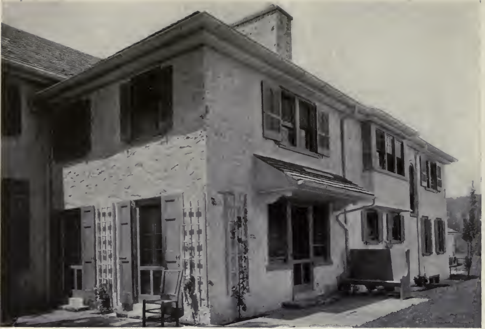
FIG. 60. BREAKFAST TERRACE AND EAST FRONT—RESIDENCE OF MRS. ALBERT B. KELLEY, RADNOR, PA. Wilson Eyre & McIlvaine, Architects.
