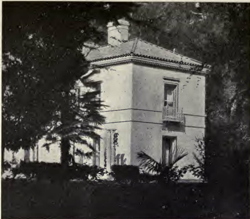
FIG. 12. RESIDENCE OF THOMAS R. BARD, ESQ., HUENEME, CAL. Myron Hunt, Architect
