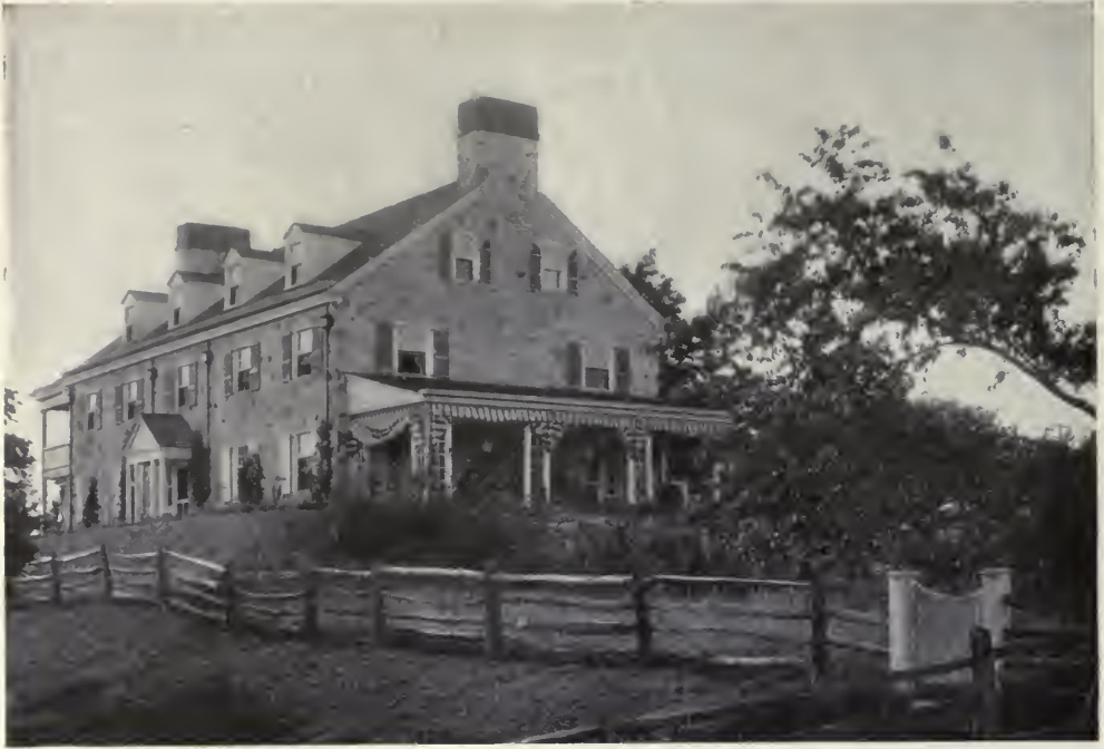
FIG. 56. SOUTH AND EAST FRONTS—RESIDENCE OF E. H. FITCH, ESQ., MEADOWBROOK, PA. Tilden & Register, Architects.
