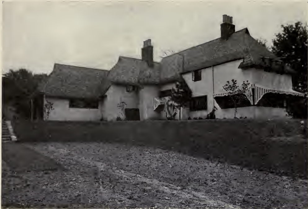
FIG. 24. RESIDENCE OF WALTER B. WALKER, ESQ., ARDSLEY, N. Y. Frank J. Forster, Architect.
