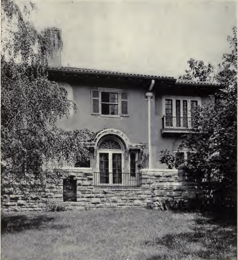
FIG. 47. GARDEN FRONT—RESIDENCE OF S. W. MOORE, ESQ., KANSAS CITY, MO. Van Brunt & Hertz, Architects.
