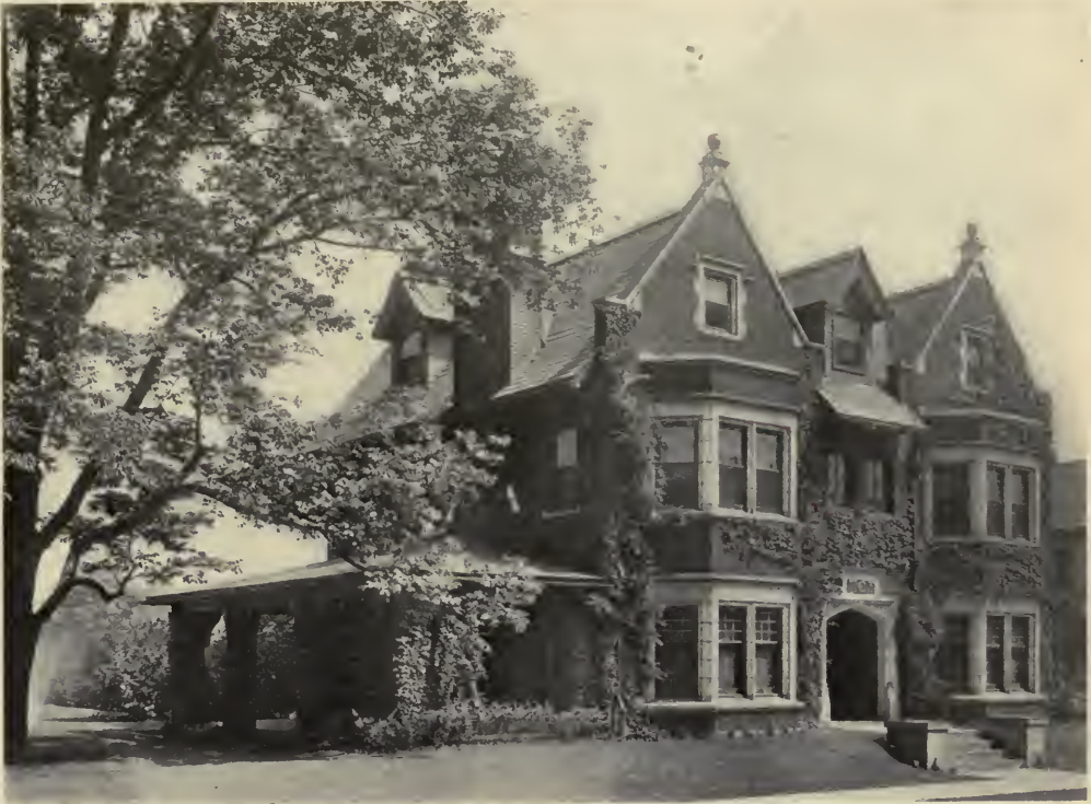
THE M. W. ACHESON, JR., RESIDENCE. Mac Clure & Spahr, Architects.
