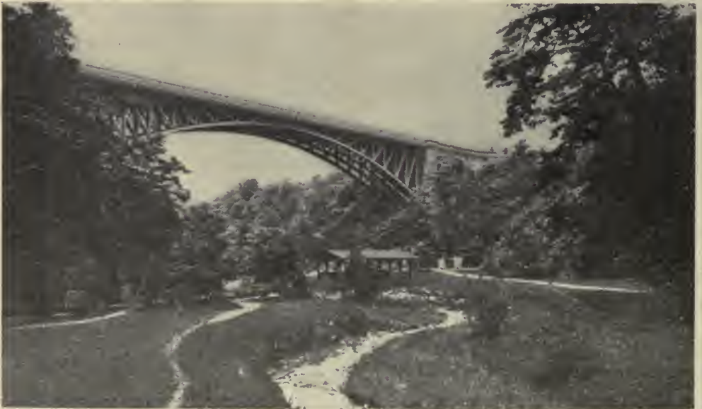
THE PANTHER HOLLOW BRIDGE.
