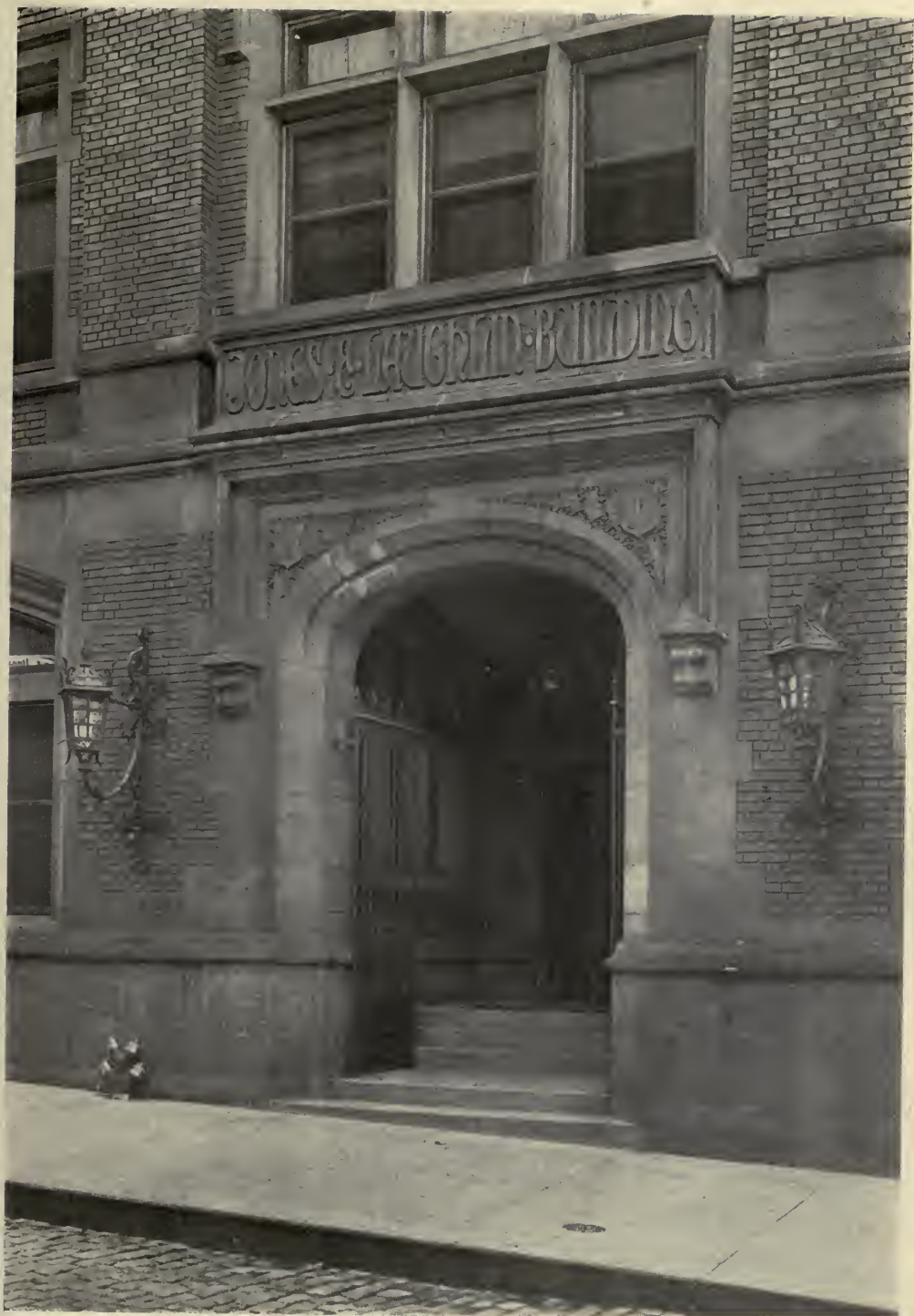
MAIN ENTRANCE—JONES & LAUGHLIN BUILDING, MACCLURE & SPAHR, ARCH'TS.
