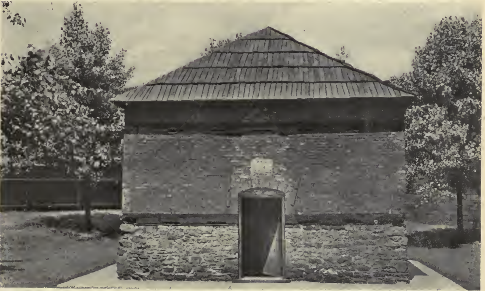
"THE BLOCK HOUSE," PITTSBURGH, A REDOUBT OF FORT PITT, BUILT 1764 (Restored).
