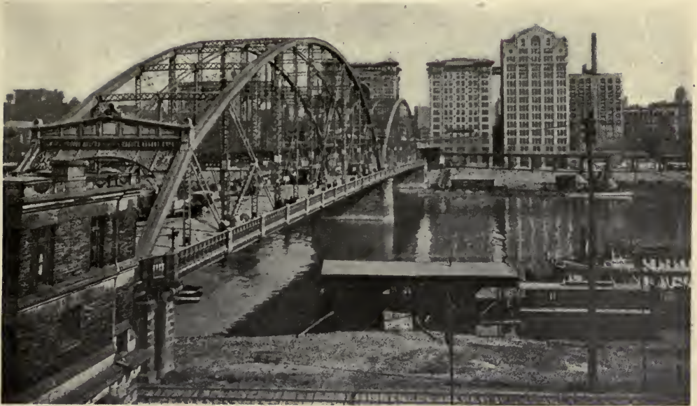
THE SIXTH STREET BRIDGE, PITTSBURGH, PA. Theodore Cooper, Engineer.
