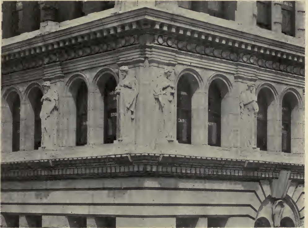
DETAIL OF THIRD STORY—FARMERS' BANK BUILDING.
