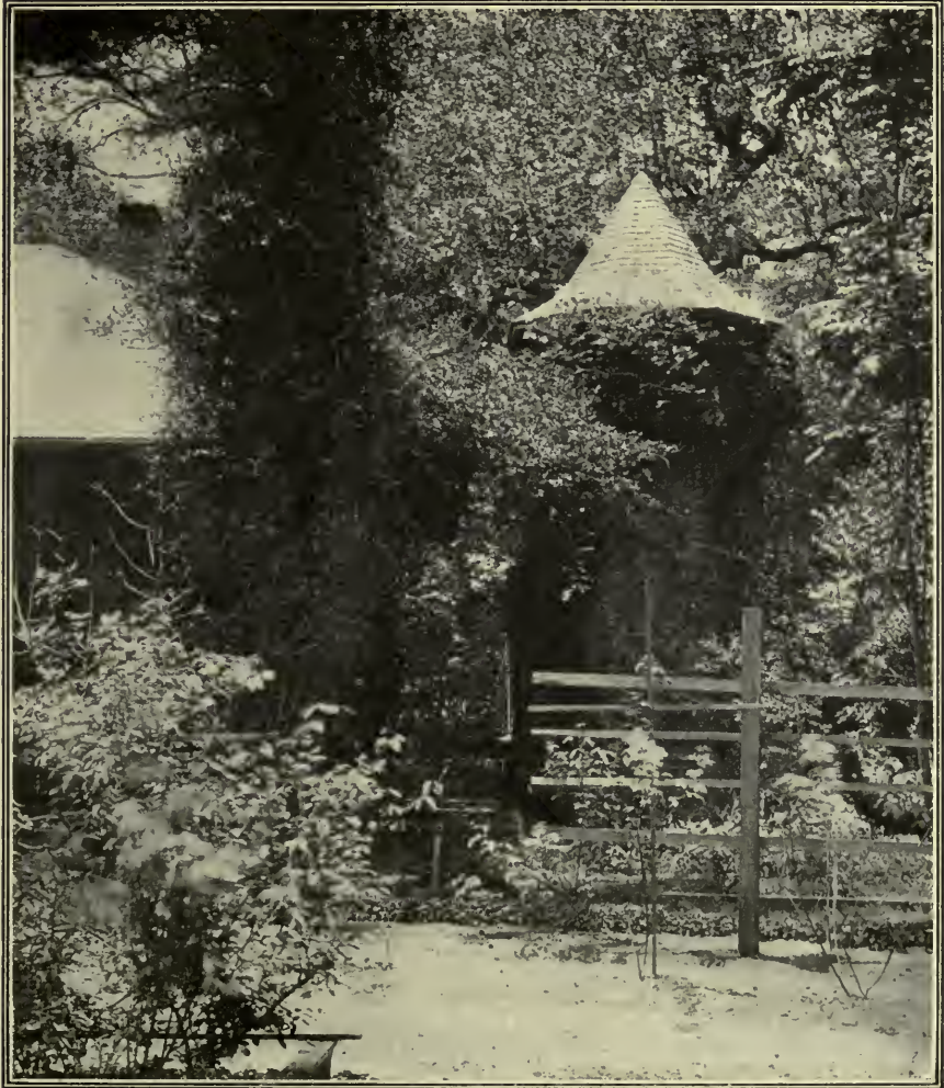
THE RAIN-WATER CISTERN.
