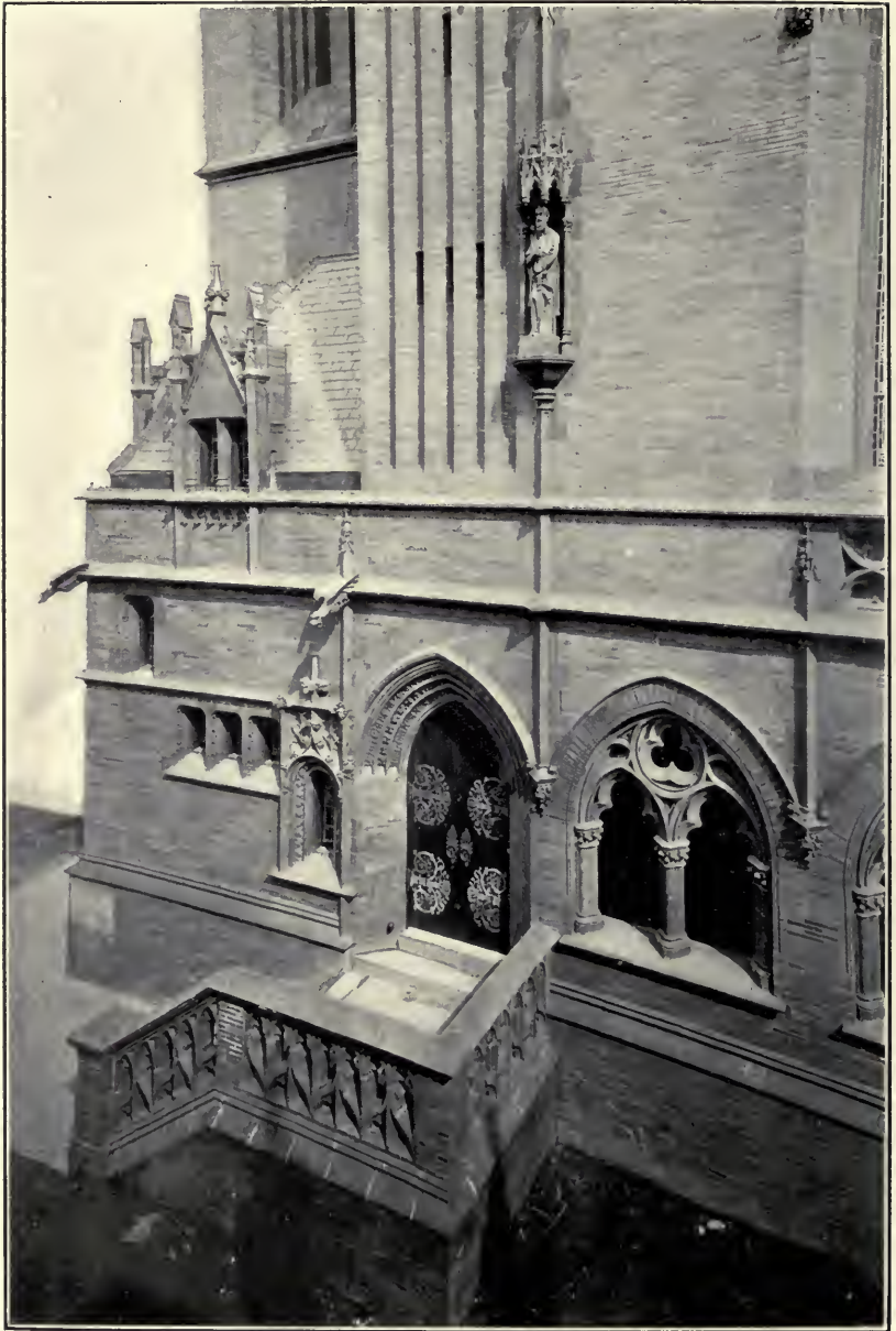
ENTRANCE TO STAIRCASE IN TOWER OF HOLY TRINITY CHURCH East 88th Street, New York City. Barney & Chapman, Architects.
