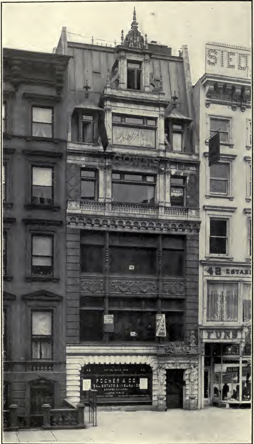
NO. 40 WEST 34TH STREET.
