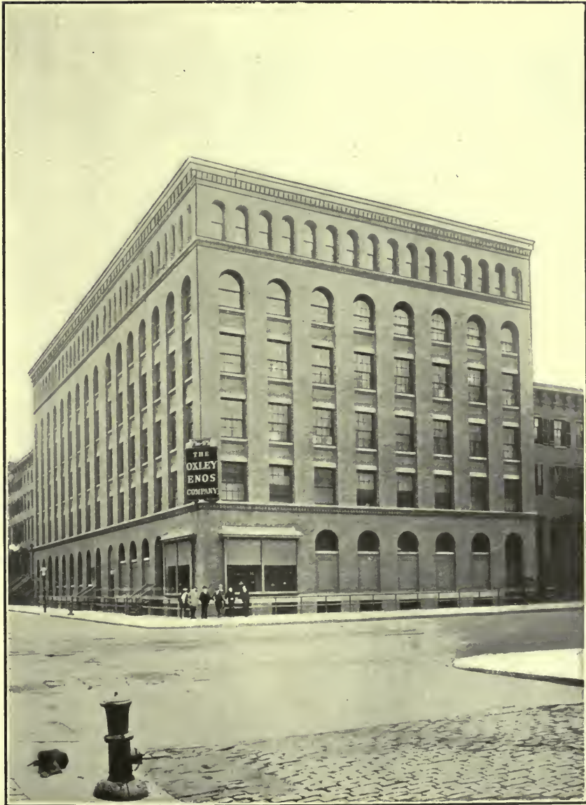
FIG. 14. FACTORY AT S. E. COR. OF 16TH ST. AND 7TH AVE. New York City. Clinton & Russell, Architects.
