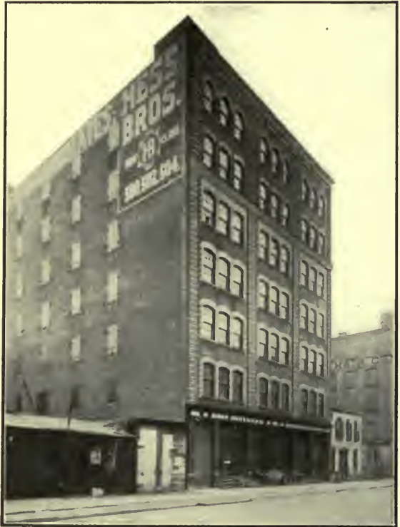
FIG. 13. NO. 500 WEST 30TH STREET. New York City. Romeyn & Stever, Architects.
