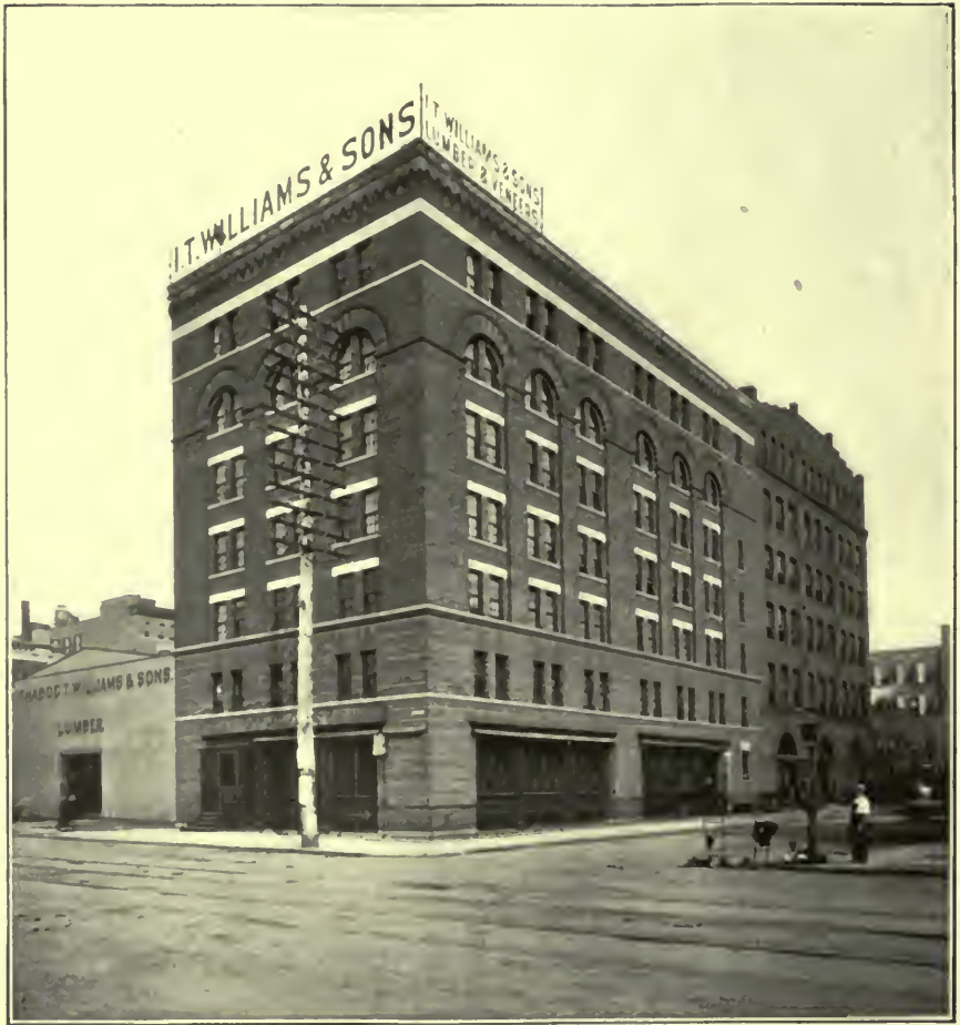
FIG. 10. WAREHOUSE OF I. T. WILLIAMS & SONS. 25th Street and 11th Avenue, New York City.
