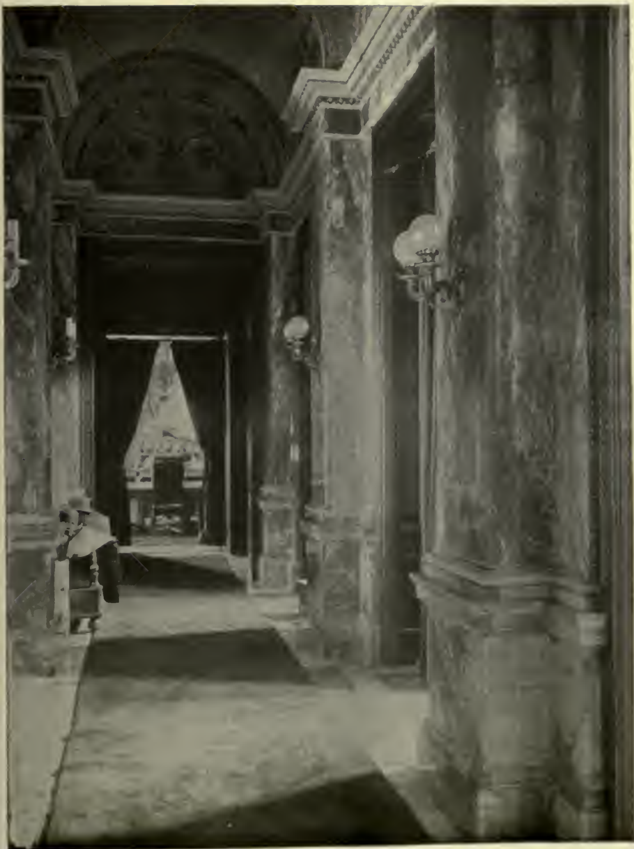
HOUSE, SOUTHEAST CORNER FIFTH AVE. AND FIFTY-SEVENTH ST. Entrance Corridor.
