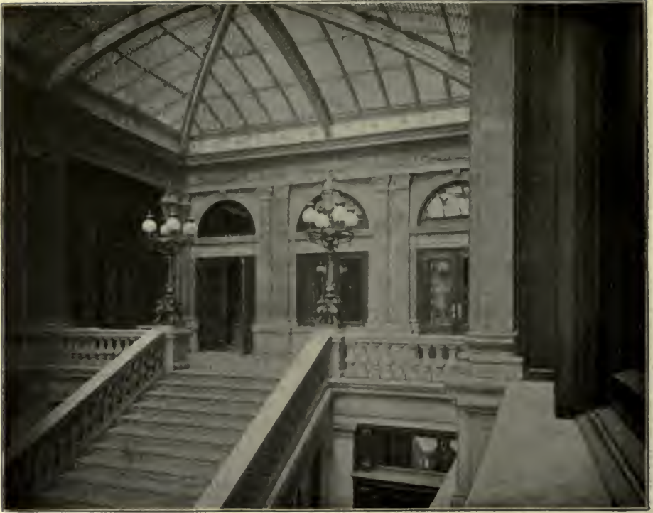
STAIRWAY OF THE MILLS BUILDING.
