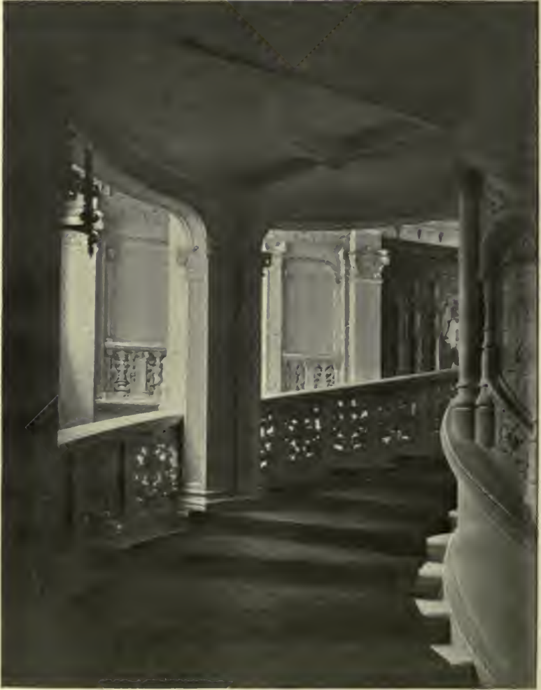
HOUSE, NORTHWEST CORNER FIFTH AVE. AND FIFTY-SEVENTH ST. Detail of Main Stairway.
