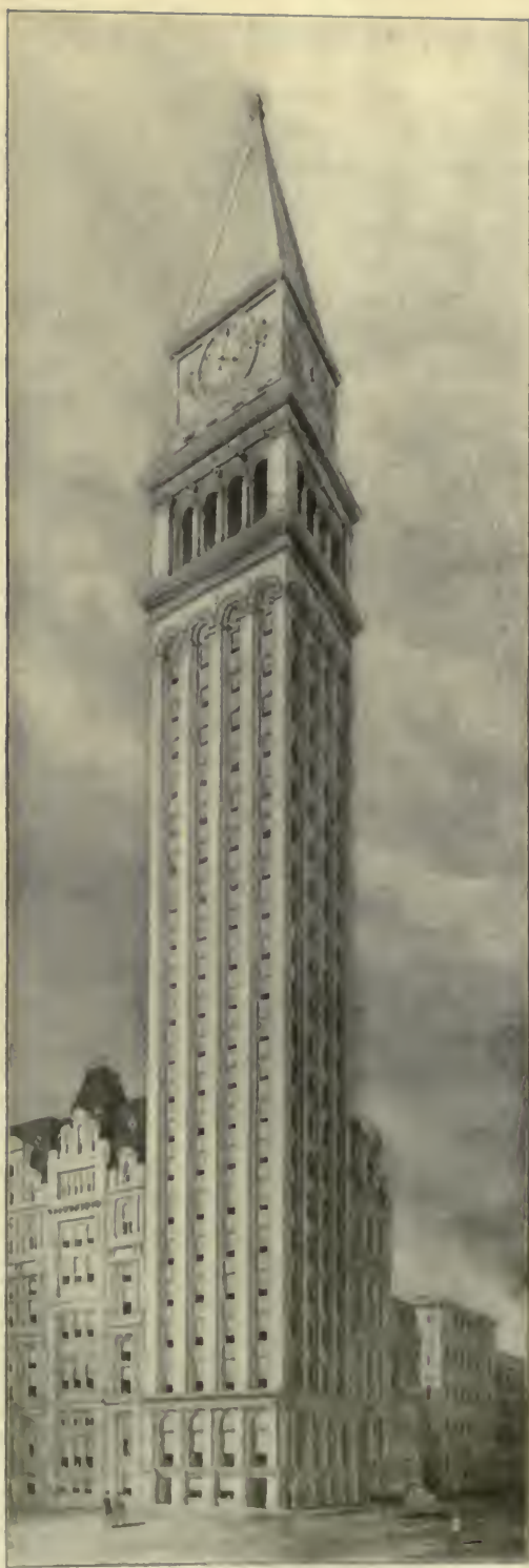
A FIVE-HUNDRED-FOOT OFFICE BUILDING.
