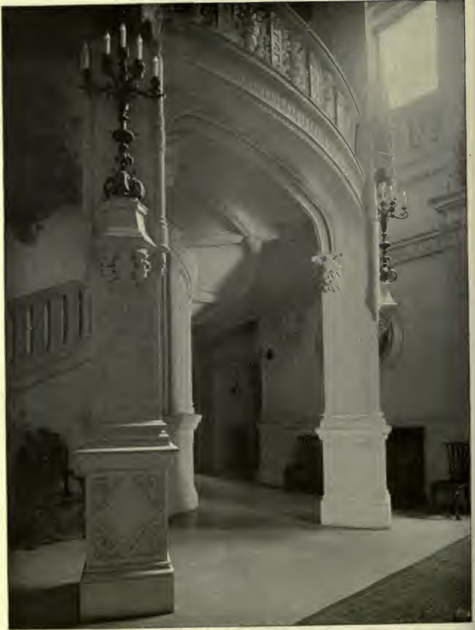
HOUSE, NORTHWEST CORNER FIFTH AVE. AND FIFTY-SEVENTH ST. Detail of Main Stairway.
