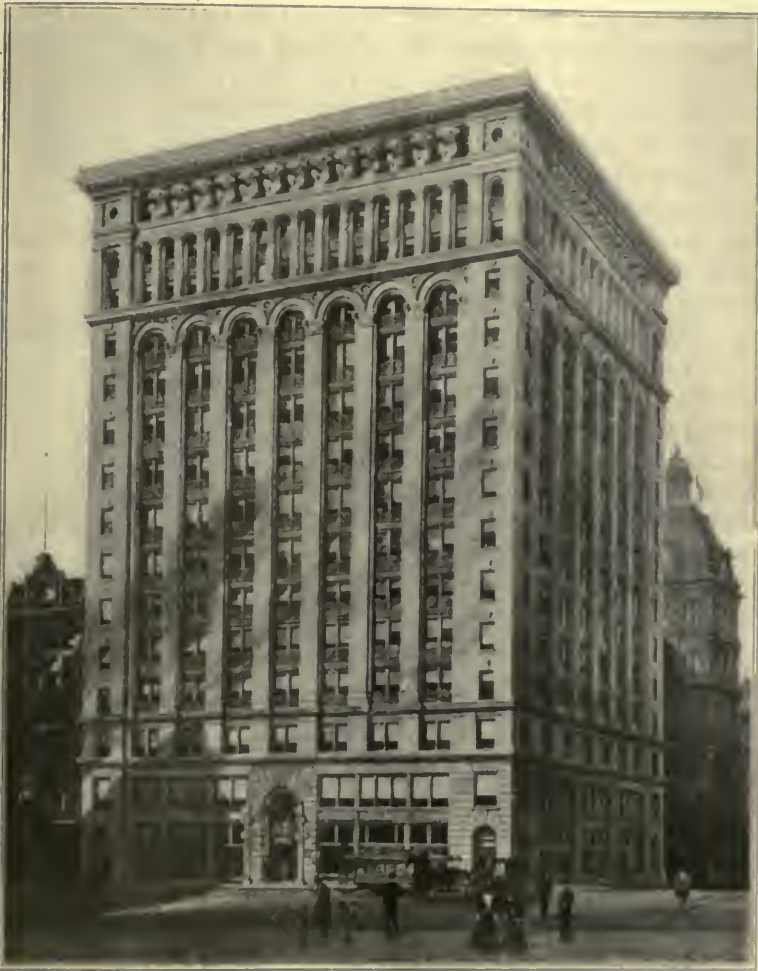
THE PARK BUILDING.
