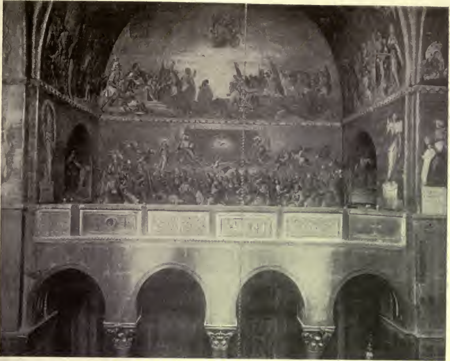
Fig. 18.—BEND IN ELEVATION, GALLERY OF ST. MARK'S, VENICE.
