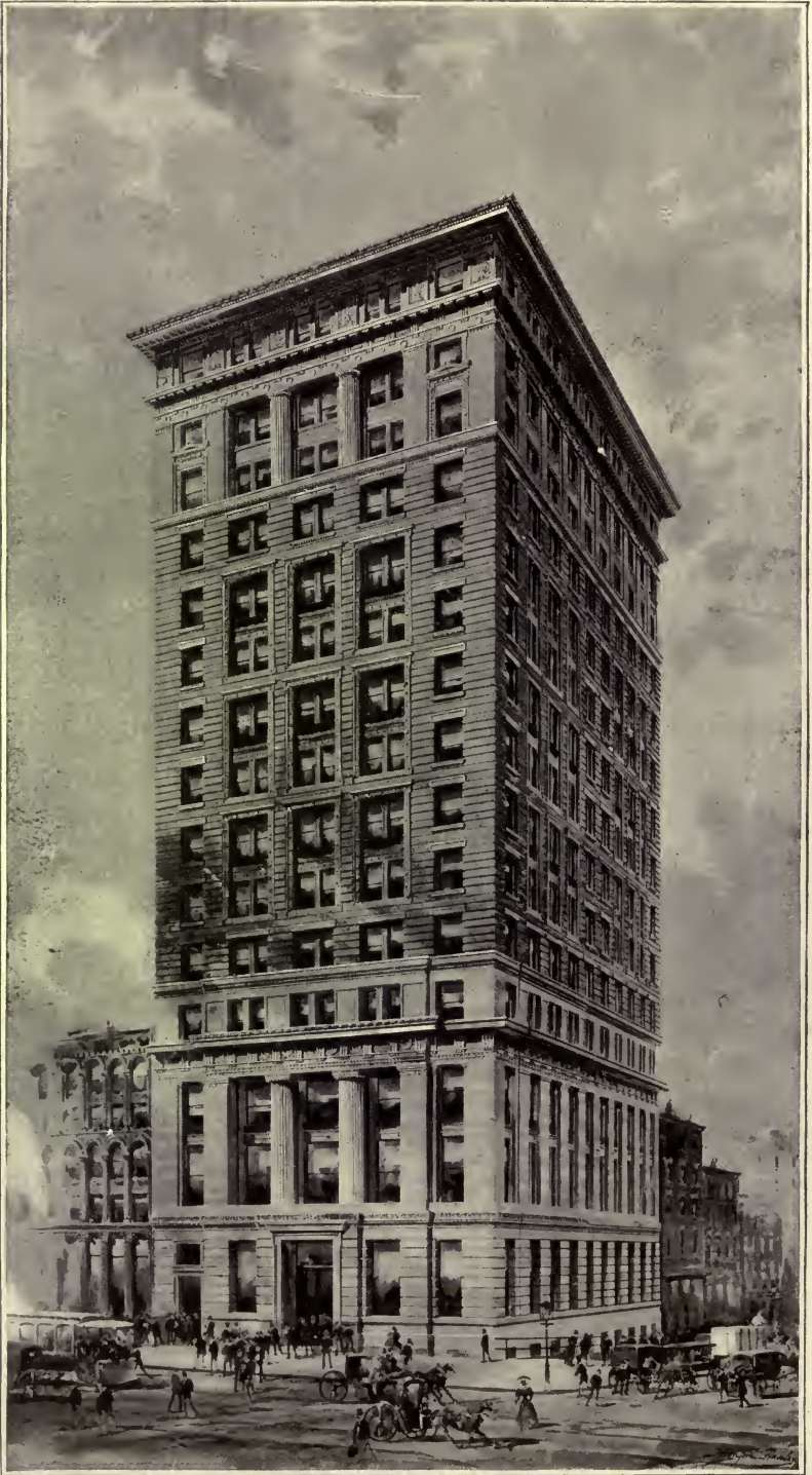
THE CENTRAL BANK BUILDING.
