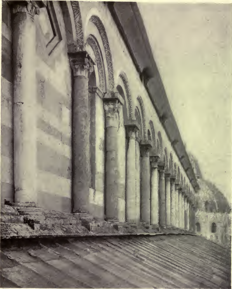
Fig. 16.—CURVE IN ELEVATION, NORTH CLERESTORY WALL, PISA CATHEDRAL.
