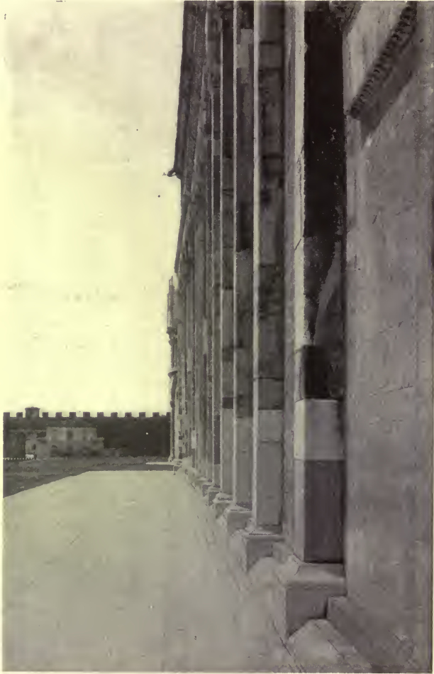
Fig. 6.—CURVE IN PLAN OF THE SOUTHWALL, PISA CATHEDRAL.
