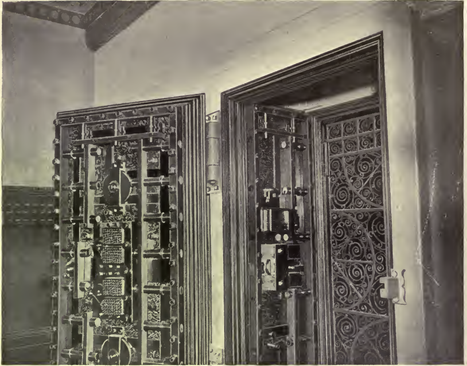
Fig. 4.—Entrance to a large vault, showing the main outer door open, one of the vestibule doors also open, and the "day-door" of ornamental scroll work closed.
