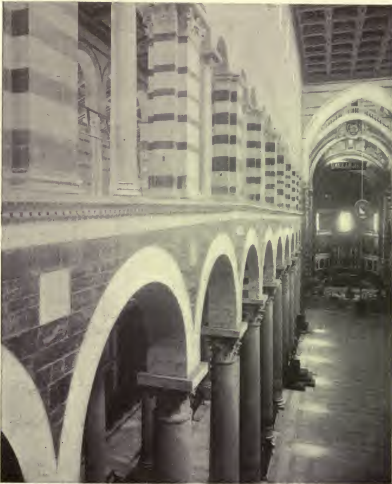
Fig. 14.—BEND IN ELEVATION, NORTH GALLERY, PISA CATHEDRAL. Brooklyn Institute Survey. Compare the section Fig. 6, Vol. VI., No. 3.
