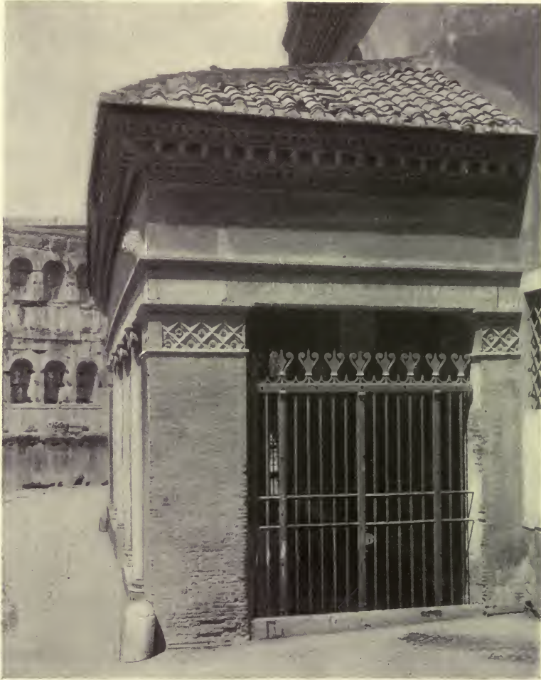
Fig. 7.—PORCH OF S. GIORGIO IN VELABRO, ROME. The cornice curves in plan; no vaulting within.
