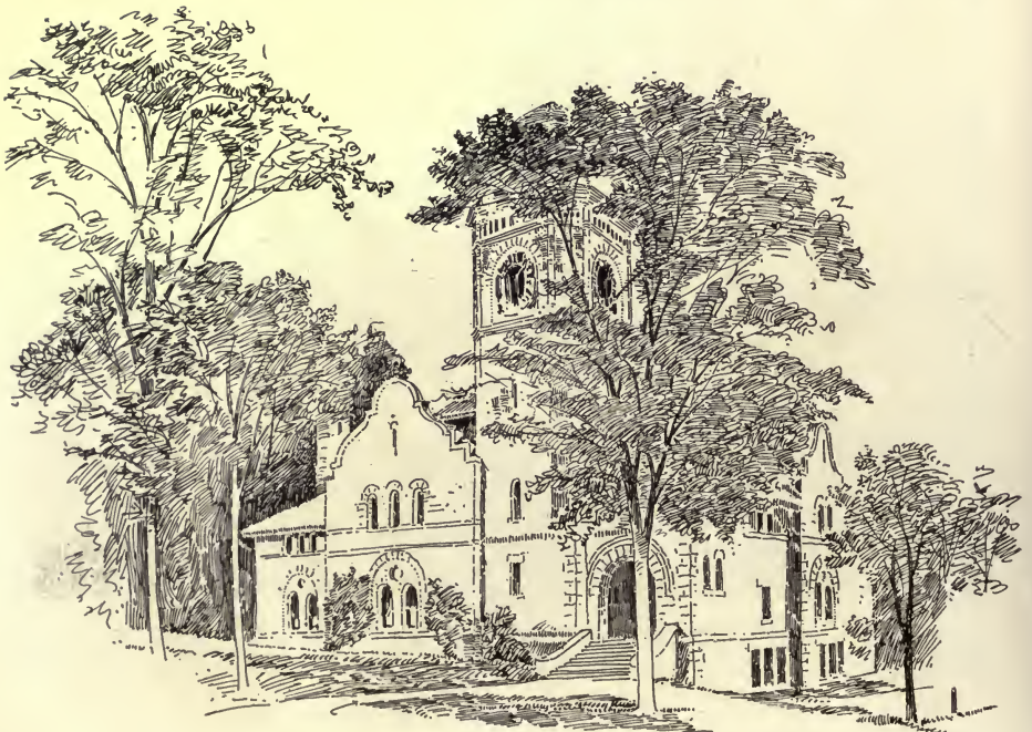
WILLIAMS COLLEGE. GYMNASIUM, WILLIAMSTOWN, MASS.
