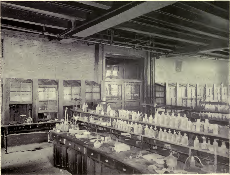
AN INTERIOR, KENT CHEMICAL LABORATORY. Henry Ives Cobb, Architect.
