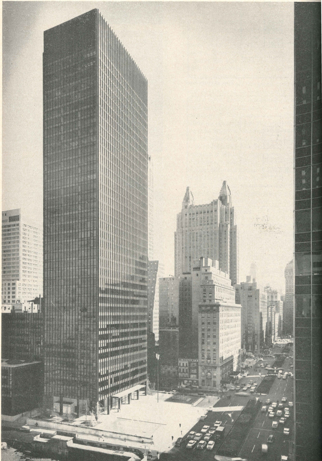
Seagram tower, flanked by low rear wings, faces Park Avenue. Plaza is raised above street level
